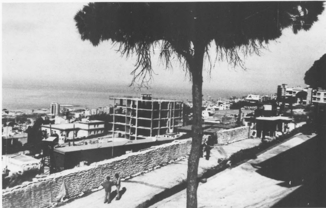
A view of the compound and remains of the bomb-damaged annex.
