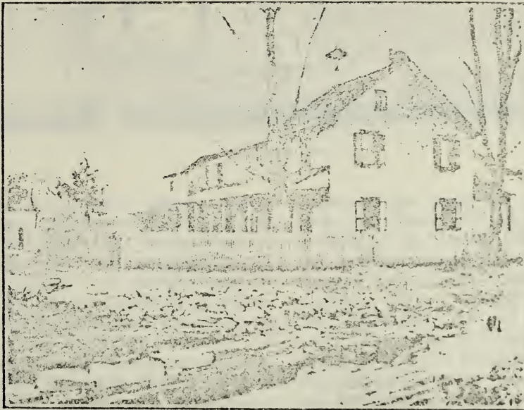
THE HOMESTEAD OF GABRIEL CARPENTER, LANCASTER CO., PA. BUILT 1730
