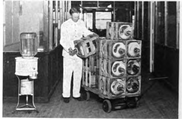
Aerated distilled water is distributed daily to office departments.
