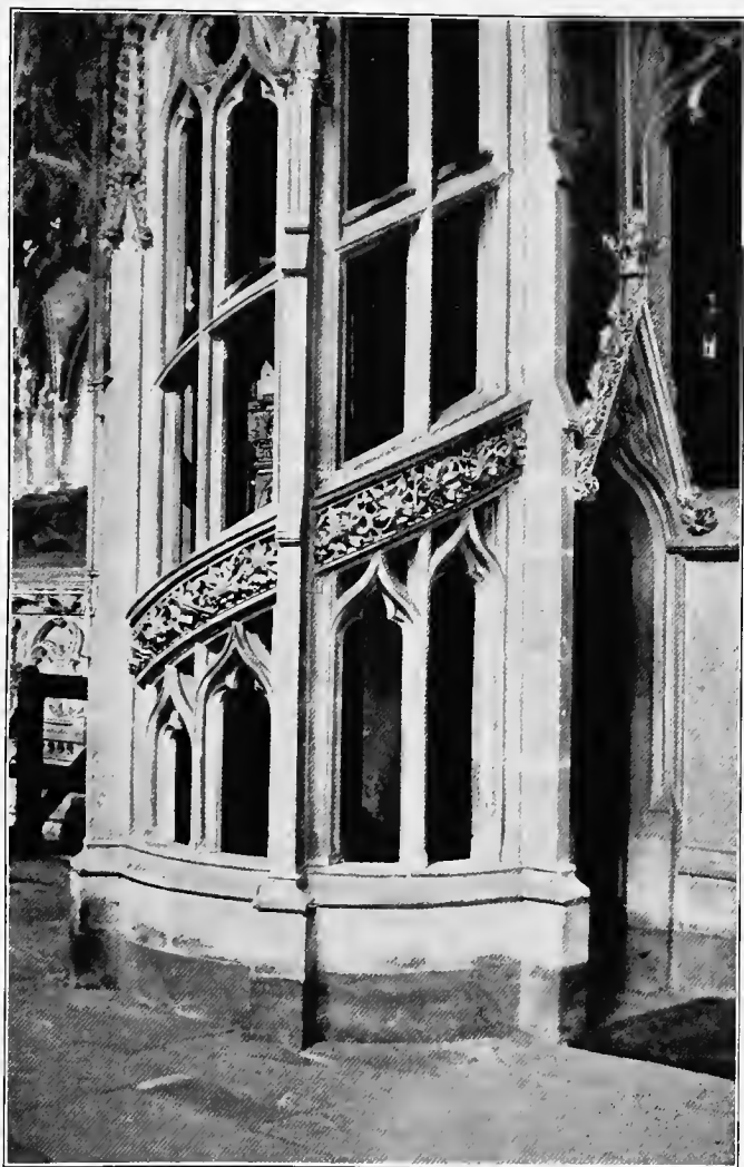
STAIRCASE TO ORGAN LOFT, ELY CATHEDRAL.
