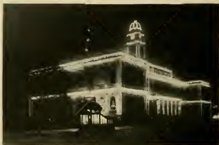
City Hall at Night
