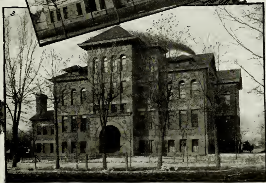
TYPICAL GRADE SCHOOL BUILDINGS IN SALT LAKE.
