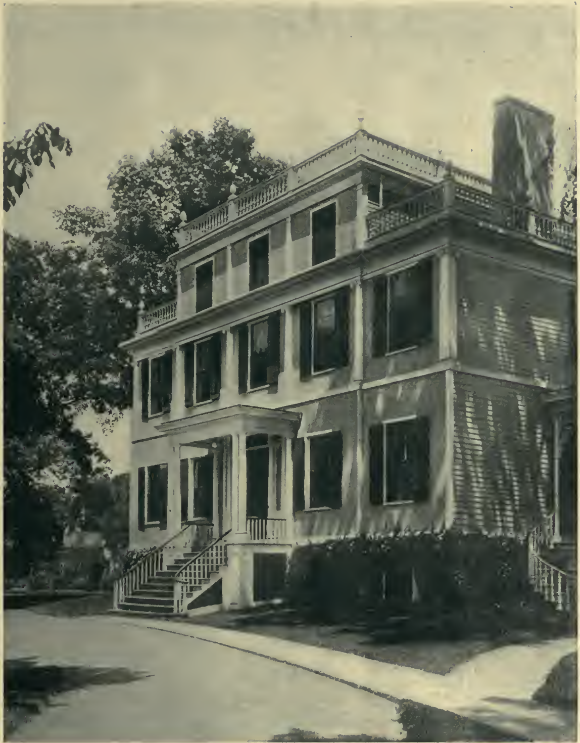
THE GRANGER HOUSE, NORTH MAIN STREET, CANANDAIGUA, NEW YORK. Front Elevation. Built circa 1816.
