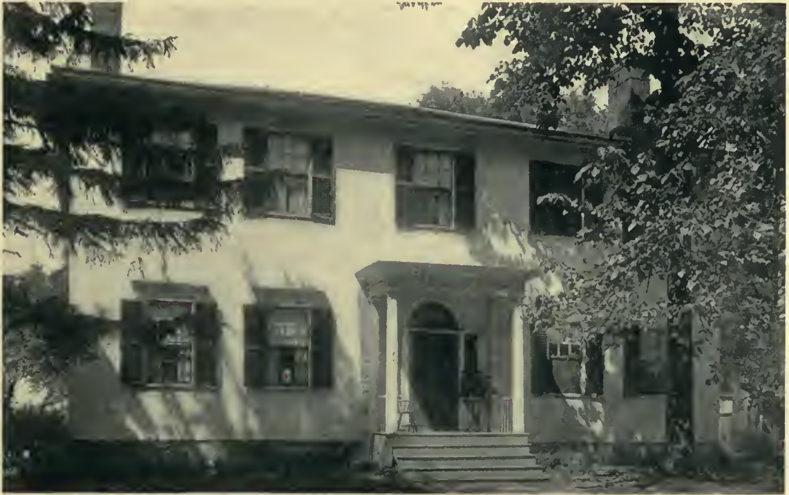
THE THOMAS BEALS HOUSE, NORTH MAIN STREET, CANANDAIGUA, NEW YORK. Built circa 1815.
