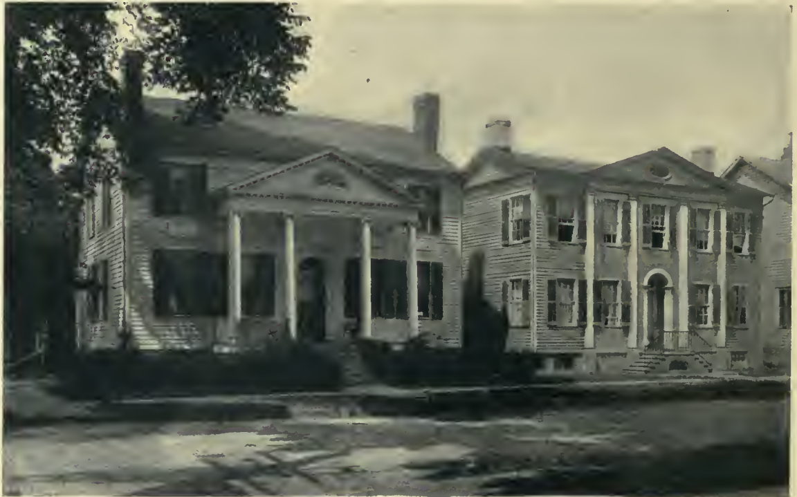
TWO HOUSES ON MILL STREET, ITHACA, NEW YORK.
