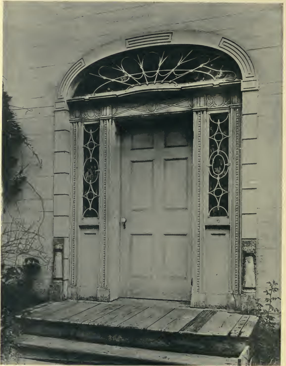
THE MILLER HOUSE, LUDLOWVILLE, NEW YORK. Detail of Doorway.
