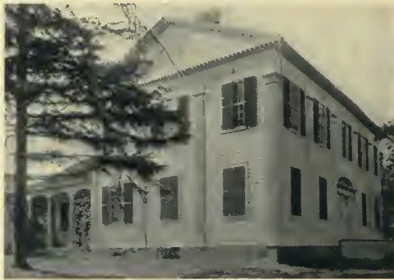
HOUSE AT VERNON CENTER, NEW YORK.
