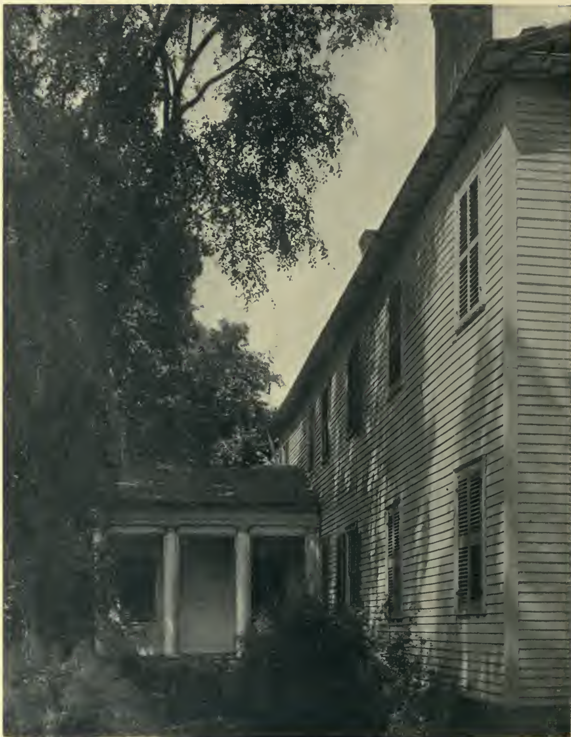
THE PHELPS HOUSE, NORTH MAIN STREET, CANANDAIGUA, NEW YORK. Detail of Side Elevation. Built circa 1813.
