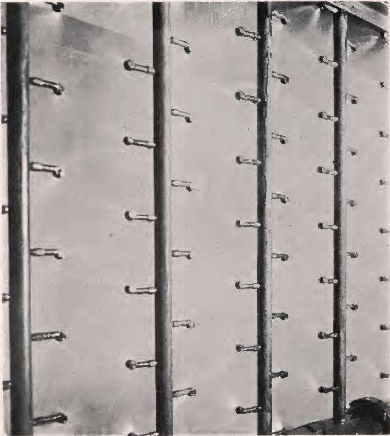
CARRIER SPRAYS IN OPERATION IN A TYPE A WASHER
