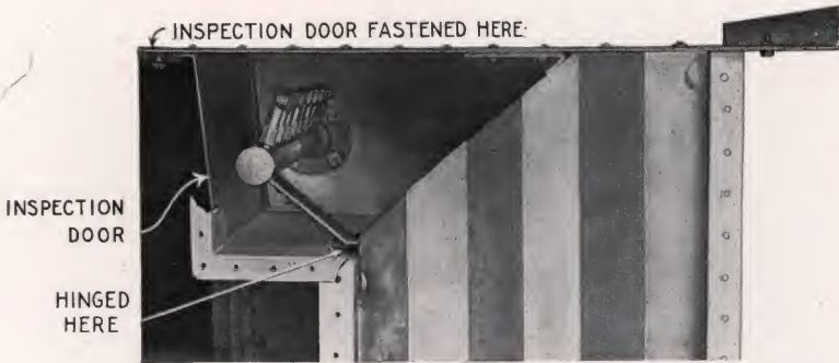
SIDE VIEW OF ELIMINATORS SHOWING FLOODING NOZZLES
