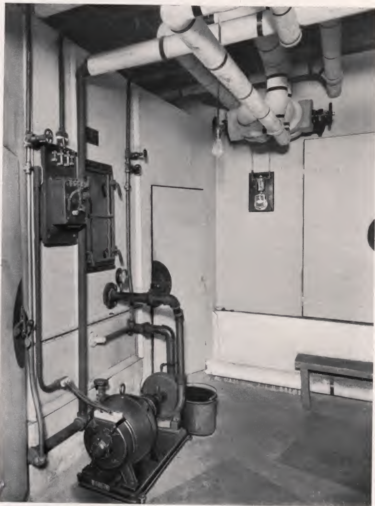
CARRIER TYPE "C" WASHER INSTALLED IN THE LEE-HIGGINSON BUILDING, BOSTON, MASS.
