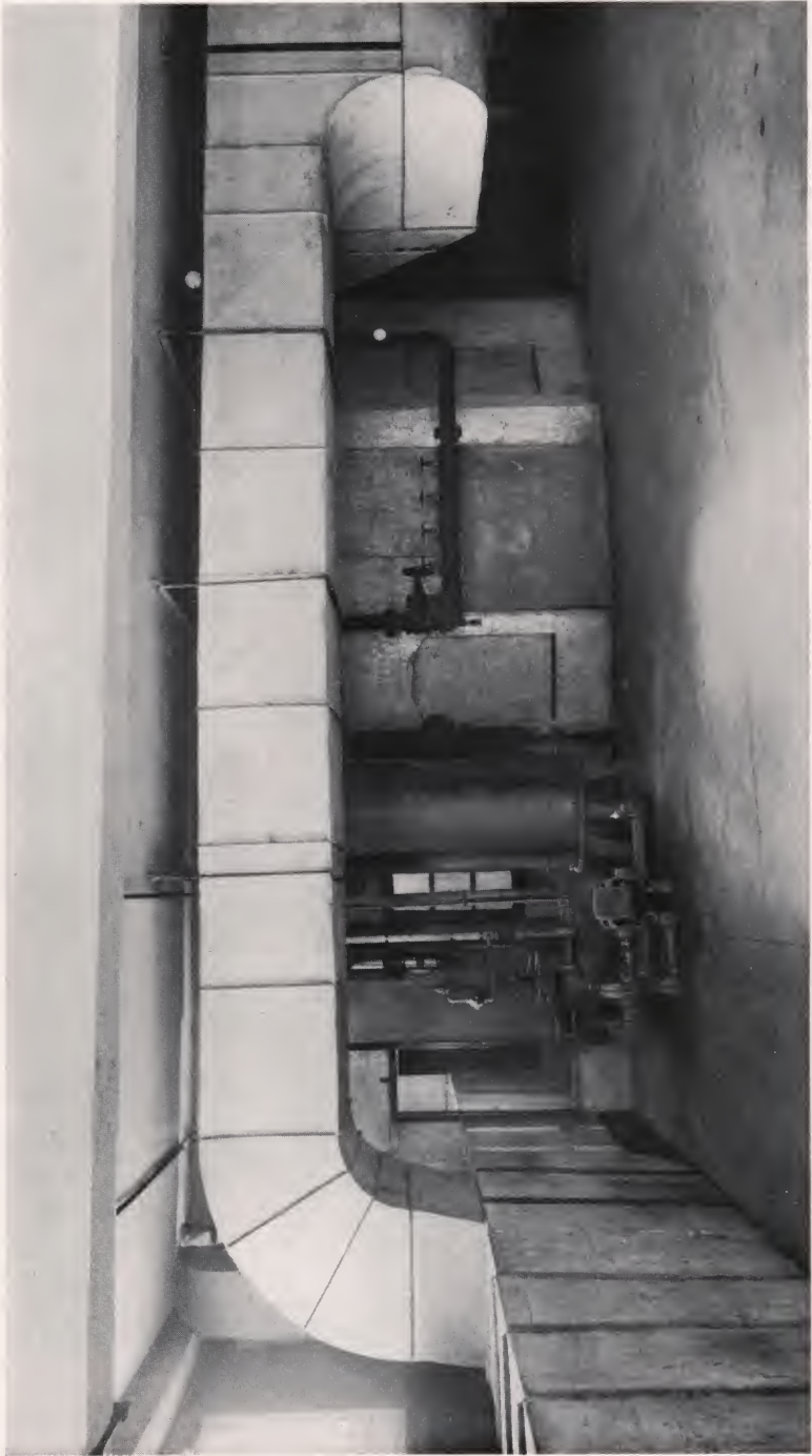
TYPE "A" WASHER WITH AUTOMATIC CONTROL INSTALLED IN THE OFFICE OF THE FORD MOTOR COMPANY, DETROIT, MICH.
