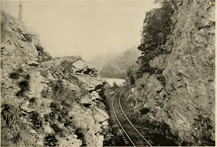
FIG. 1.—RAILROAD CUT IN CONTORTED GNEISS, ABOVE BALD FRIAR.
