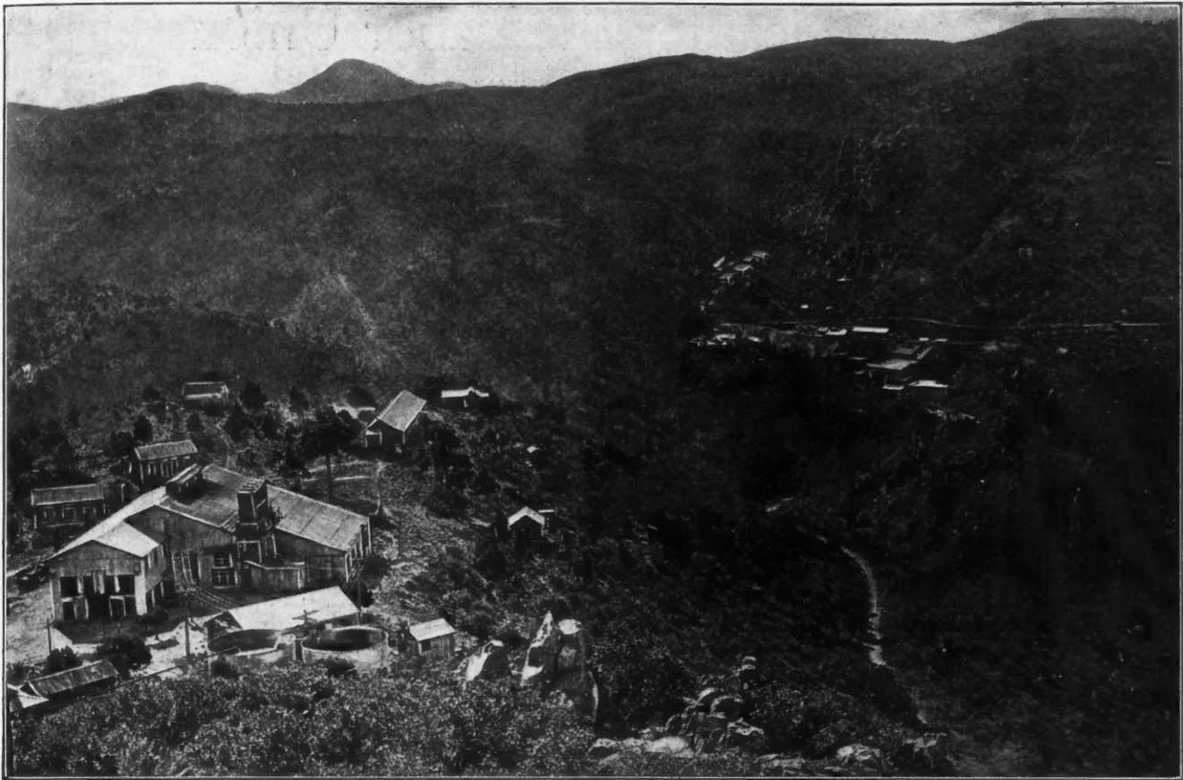
MINING AND MILLING CO. IN FOREGROUND. IN THE DISTANCE ON THE RIGHT IS SHOWN THE MOGOLLON MINES WEATHERHEAD. IN THE CANYON ON THE LEFT, PART OF THE TOWN OF MOGOLLON MAY BE SEEN
