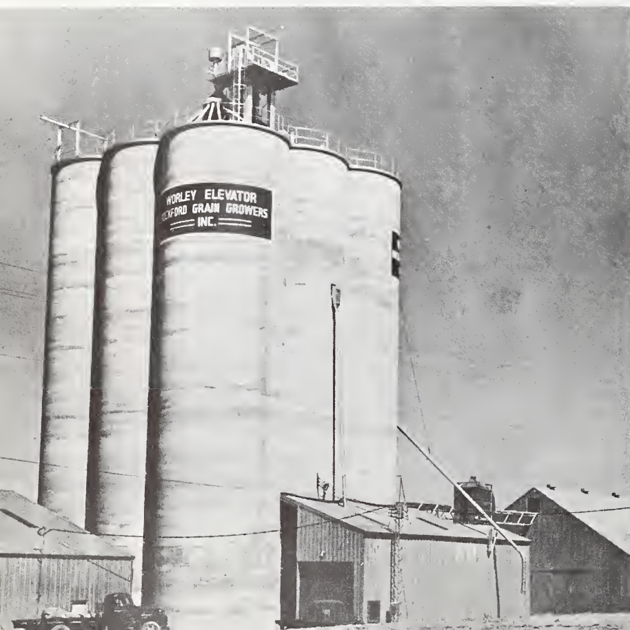
A typical country elevator station in the Pacific Northwest.
