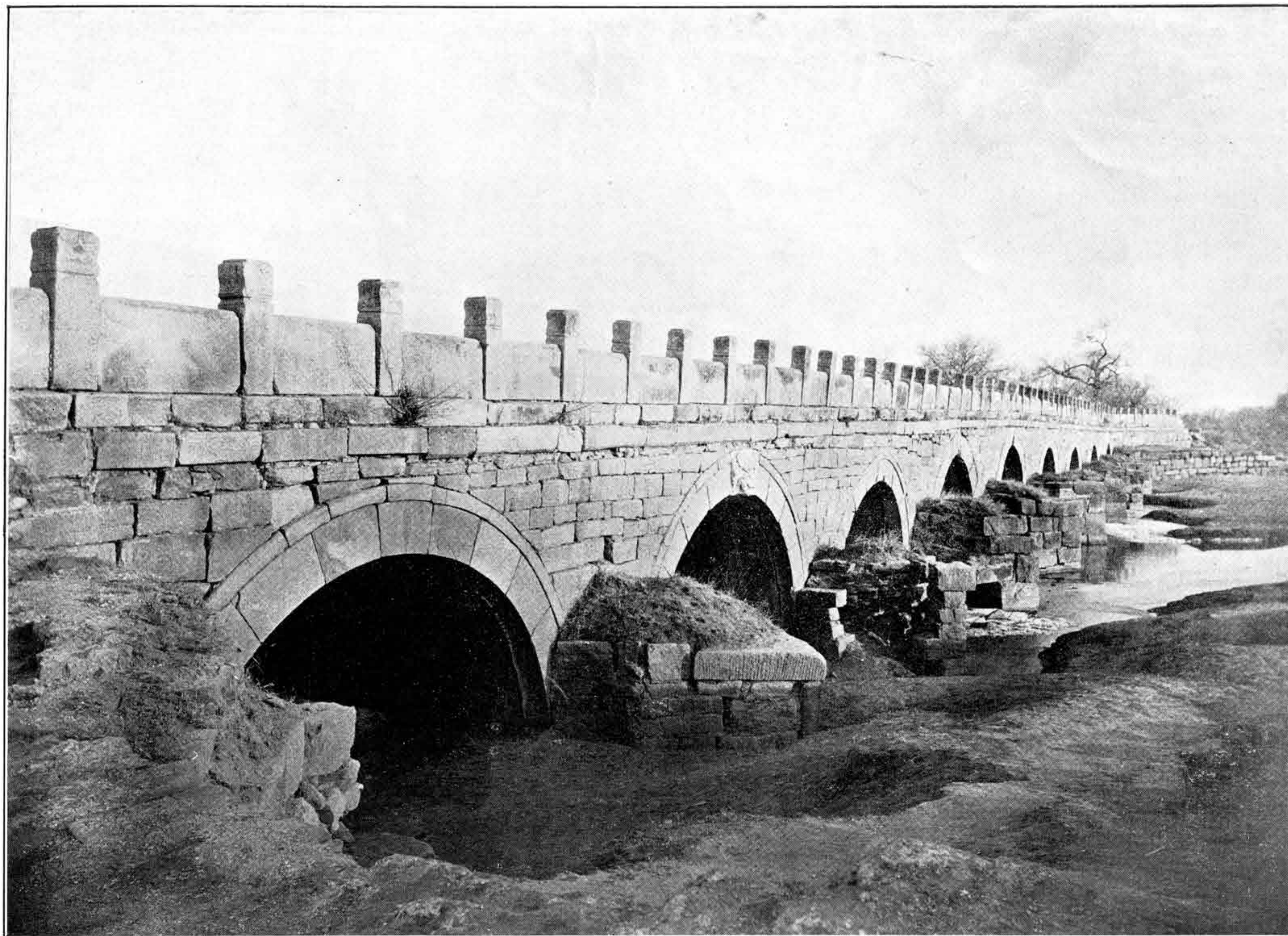
No 52. Sha-Ho-ch'iao Bridge.
