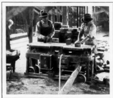
Portable Brick Cleaner and Shaper in Operation; a Revolving Unit Knocks Off Scale and Mortar
