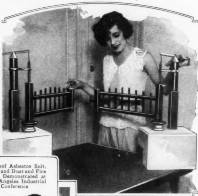
An Inventor's Model of His Railroad Crossing Gates, Which Work by Gravity and Eliminate the Services of an Attendant; Transportation Offers a Good Field for New Ideas
