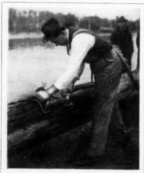
Planing a Big Log by Air-Driven Smoother; the Bark Is Quickly Taken Off without Damaging Wood
