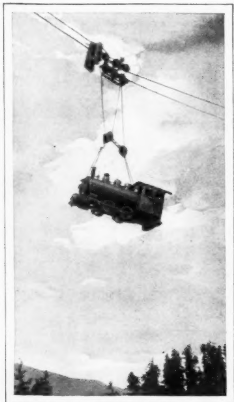
Where a Locomotive Takes the Air; Swinging Work Engine across Canyon on Steel Cables
