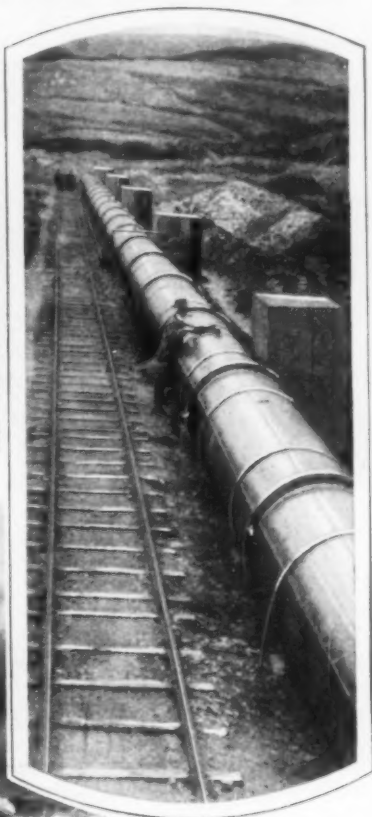
Reading the Record of the Speed of the Explosion. Connecting Instruments Used in the Big Test Tube and the Mouth of the Chamber at the Instant the Explosion Occurred
