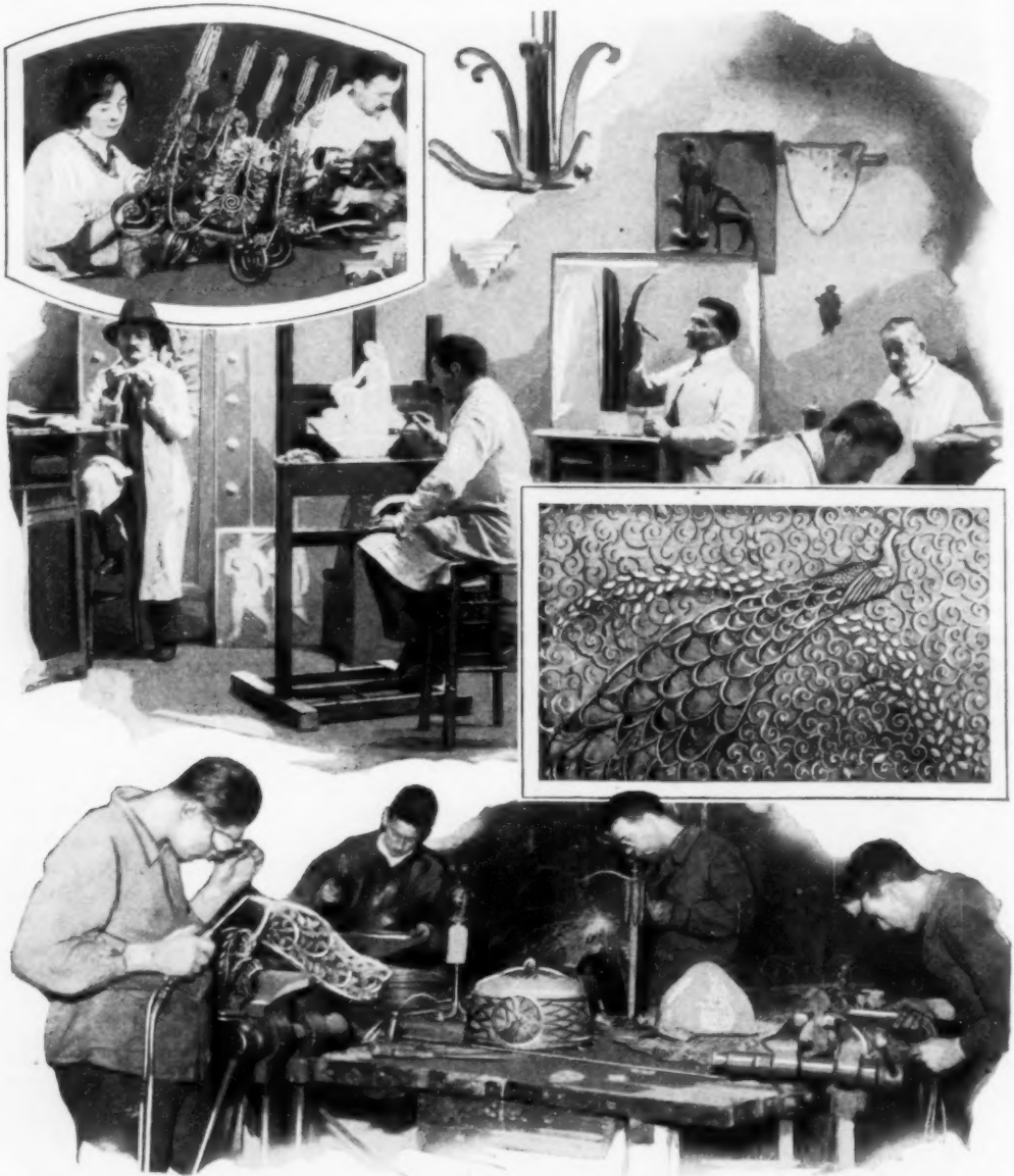
Below, Welding Delicate Pieces of Iron for Chandeliers; Center, Making Designs and a Fire Screen; Top, Left, Giving Iron Appearance of Old Bronze
