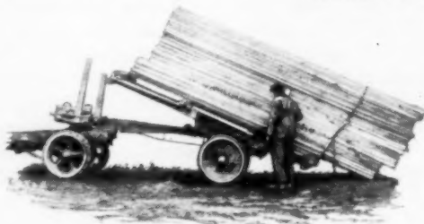
Unloading Lumber as One Unit
