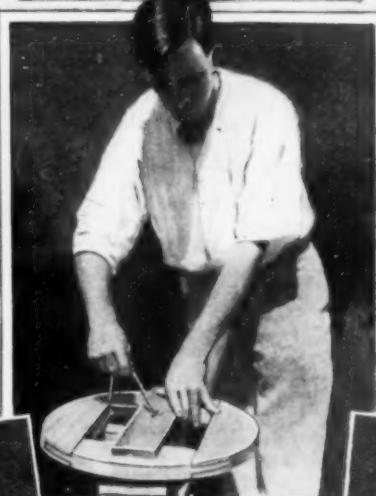
Locating Center of Wheel on Temporary Spokes
