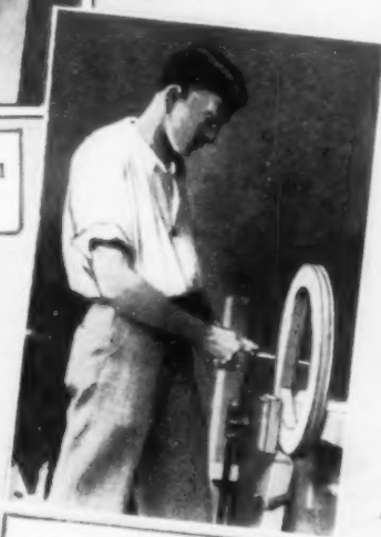
Sawing Out Inside of Rim with Keyhole Saw
