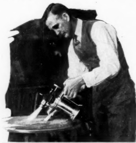
Greater Safety Is Claimed for This Blowtorch with Automatic Valve; It Burns Gasoline or Kerosene
