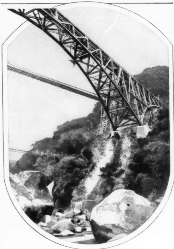
One End of the Lofty Steel Bridge Recently Built in Japan; It Is 450 Feet Long and Spans a Gorge 500 Feet Deep
