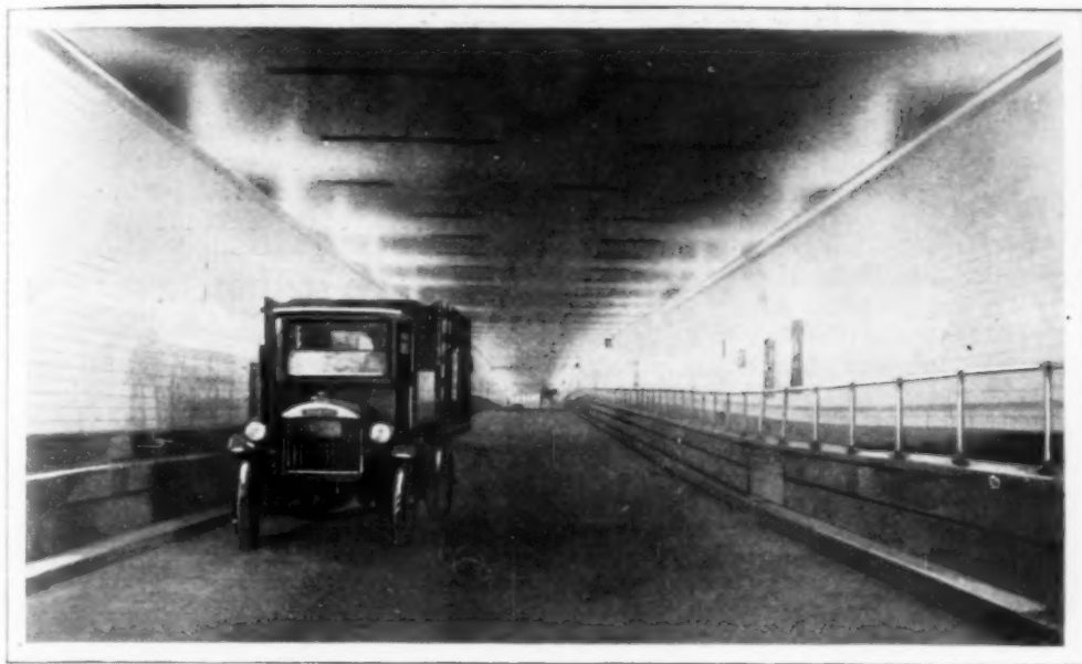
Interior of One of the Twin Tubes under the Hudson, Showing the Ventilation Ducts in the Ceiling, and the Sidewalk at the Side for the Police Who Regulate the Traffic
