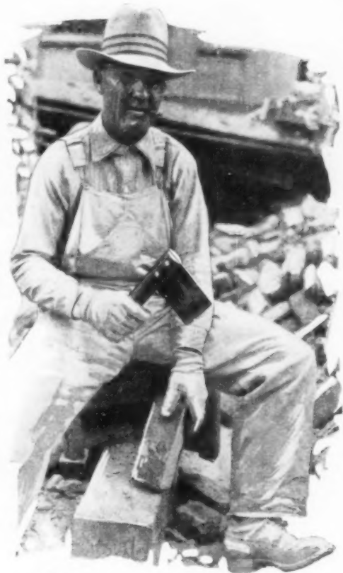
Auto-Wheel Spoke and Piece of Steel Plate Make Tool for Removing Mortar from Bricks
