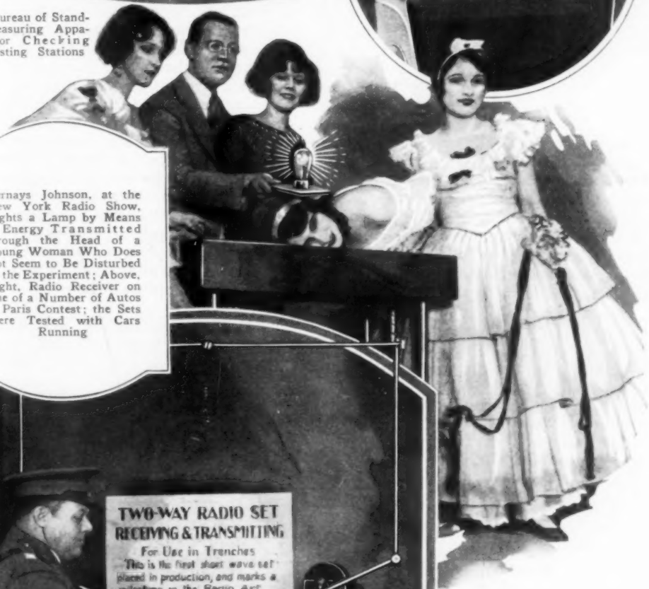
Left, Captain Autrey, of the U. S. Signal Corps, with One of the Latest Types of Radio-Receiving and Transmitting Sets Designed for Use in Trenches; These Two-Way Short-Wave Sets Are Portable and Mark an Advanced Step in Radio Communication as Applied to Field Use under War Conditions
