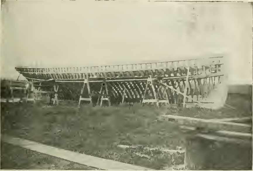
A SHIP ON THE WAY READY FOR PLANKING.
