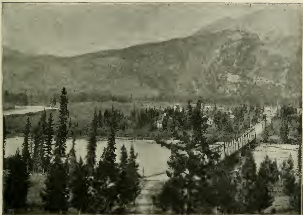
BOW RIVER BRIDGE, BANFF.
