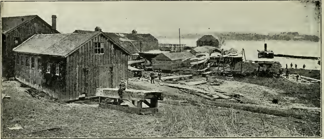
A PORTION OF ROBERTSON BROS.' SHIPBUILDING YARD.
