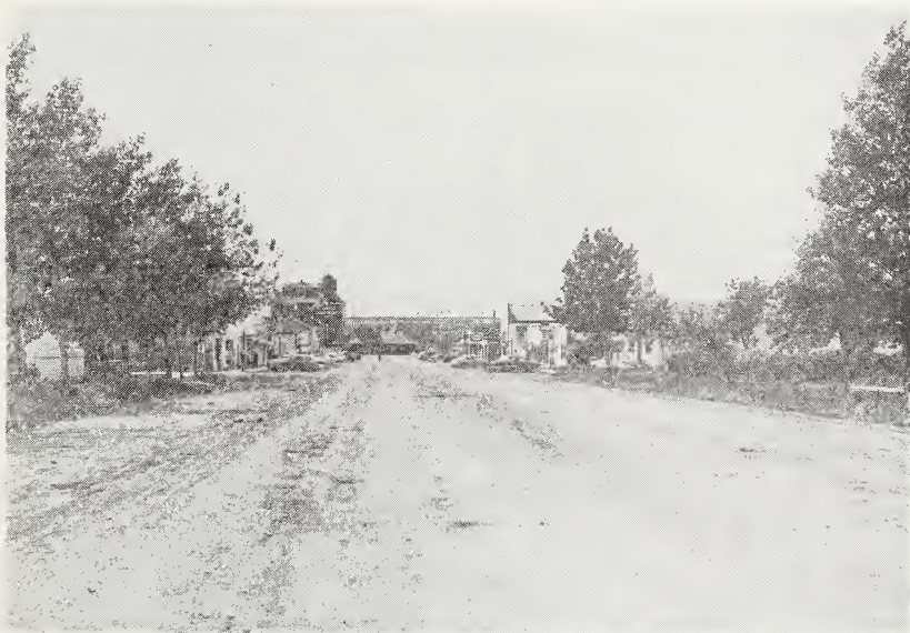
Broad Main Street is attractively lined with trees
