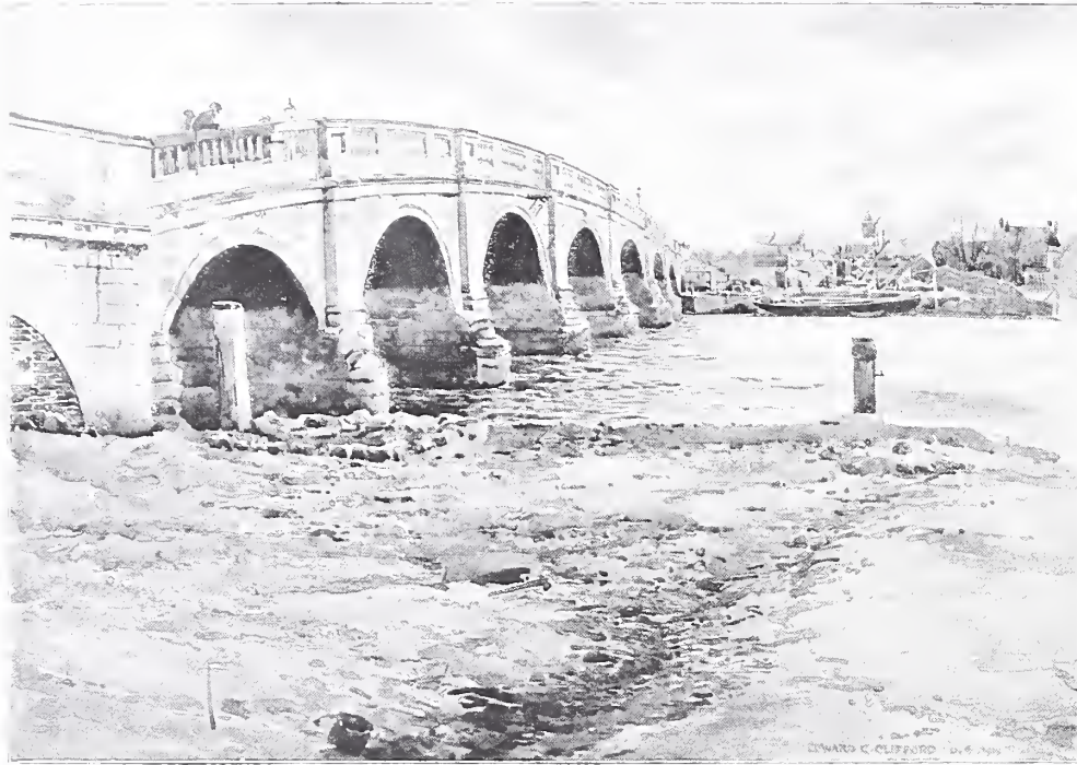
The Brentford End of the Bridge.
