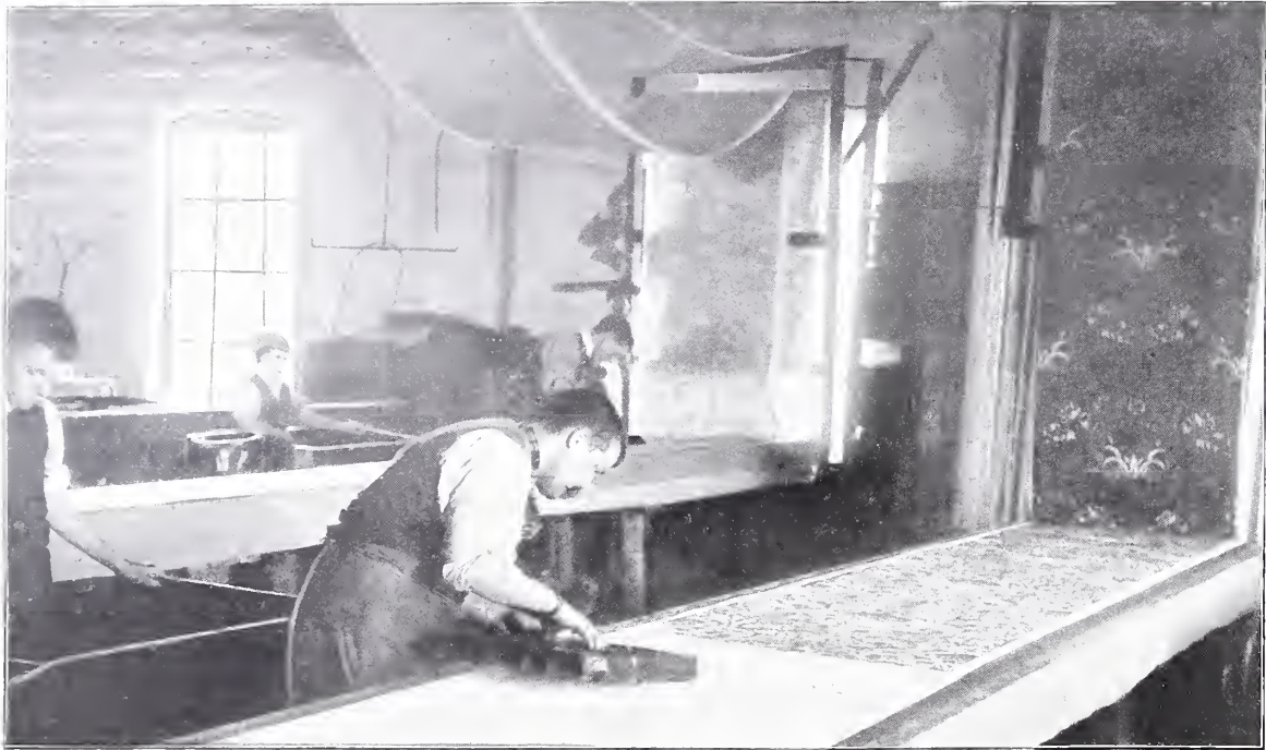
Hand Block Printing—Laying first colour.
