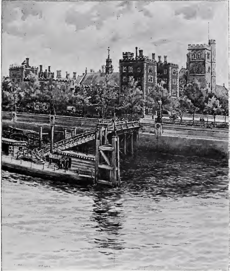
Lambeth Palace from Lambeth Bridge.
