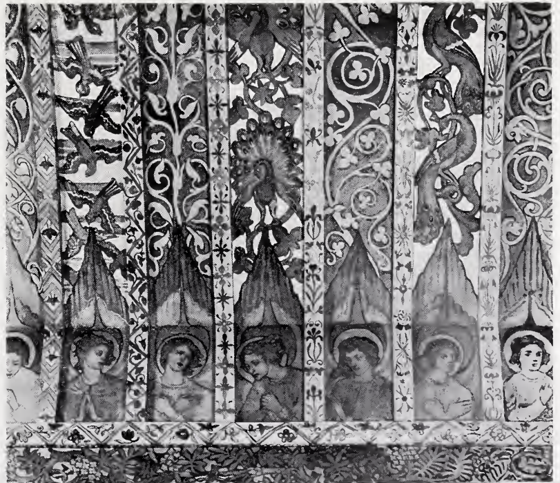
Detail of Roof in North Aisle, Catholic Apostolic Church, Edinburgh.
