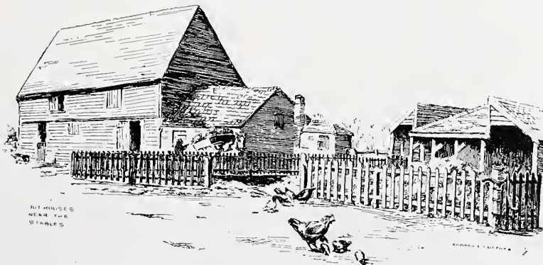
Outhouses near the Stable, Fulham Palace. A drawing by Edward C. Clifford, R.I.
