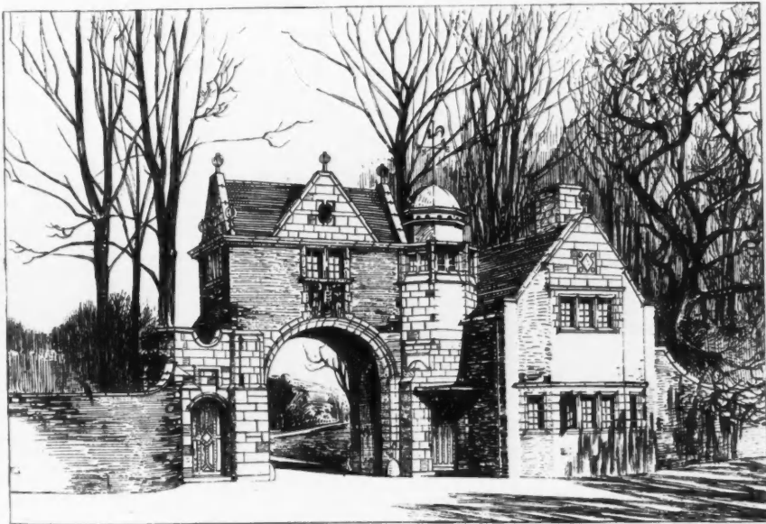
1754. Lodges at Lea Park, for Whitaker Wright, Esq., PAXTON WATSON, A.R.I.B.A., Architect. (For Plans, see p. 31.)
