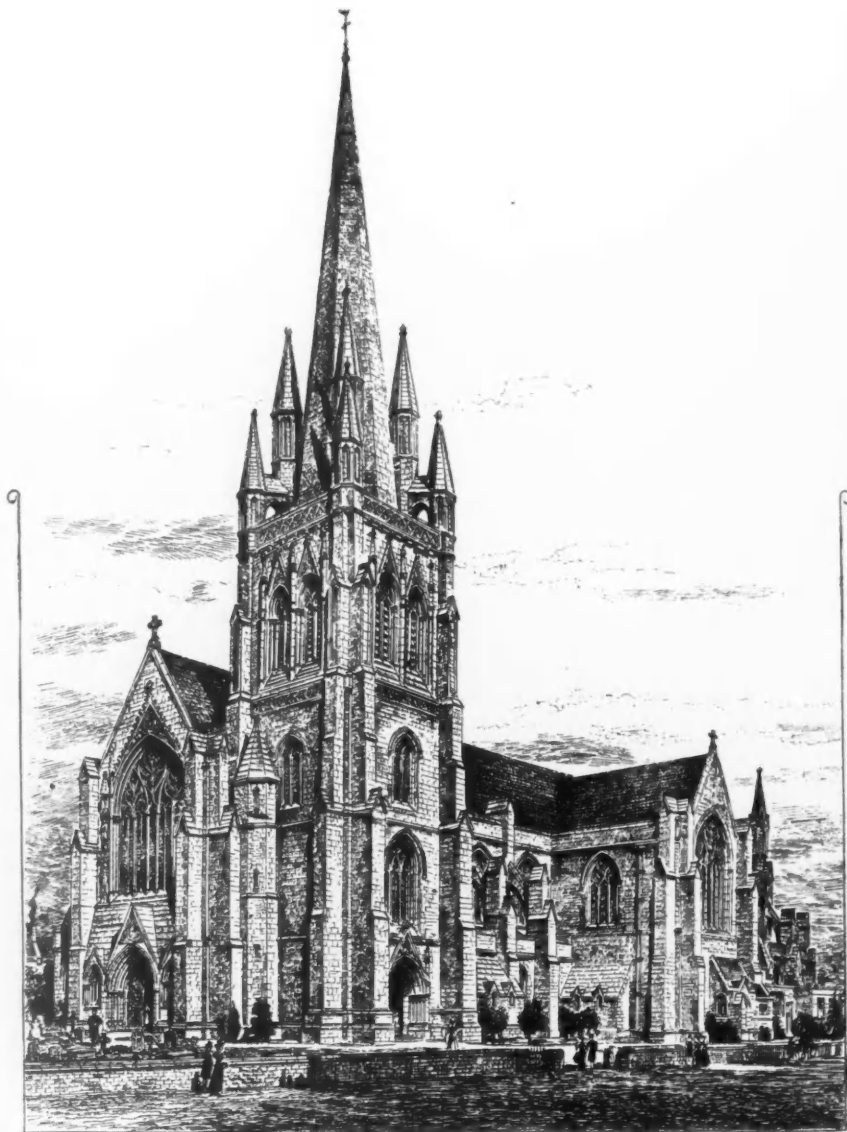
St. Alban's Church, Blackburn, EDWARD GOLDIE, Architect.
