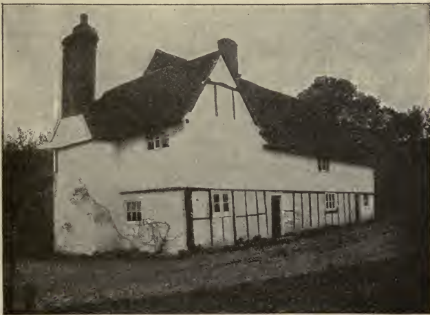
An old farmhouse, near Wheathampstead, Hertfordshire
