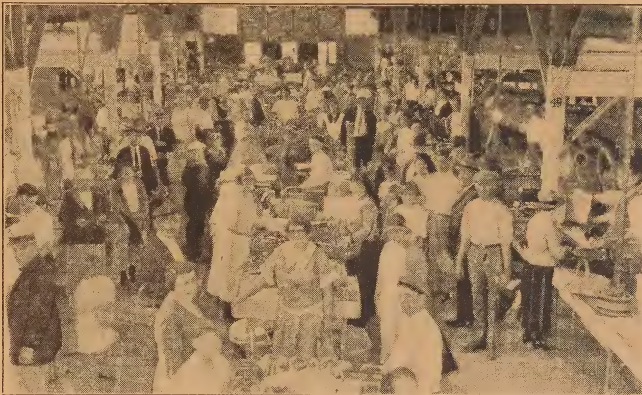
The interior of one of the Binghamton market houses. In September there were 933 farmers on the market
