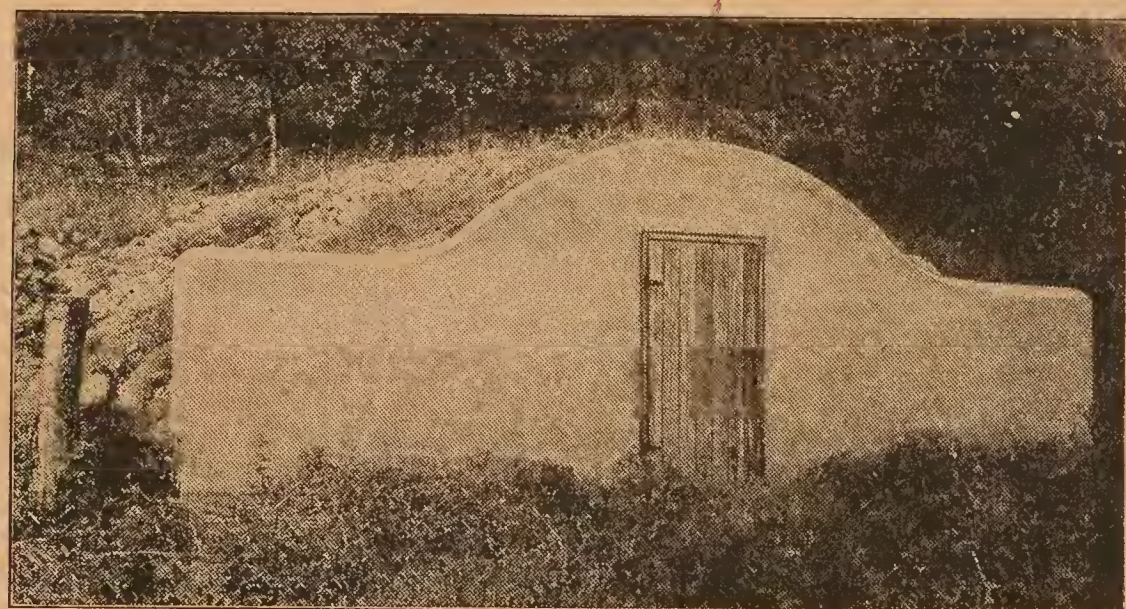
Success in storing farm produce, such as potatoes, depends a great deal on the manner in which the storehouse or cellar is constructed. This house is so built that a bank of earth is taken advantage of, concrete adding to its permanence.
