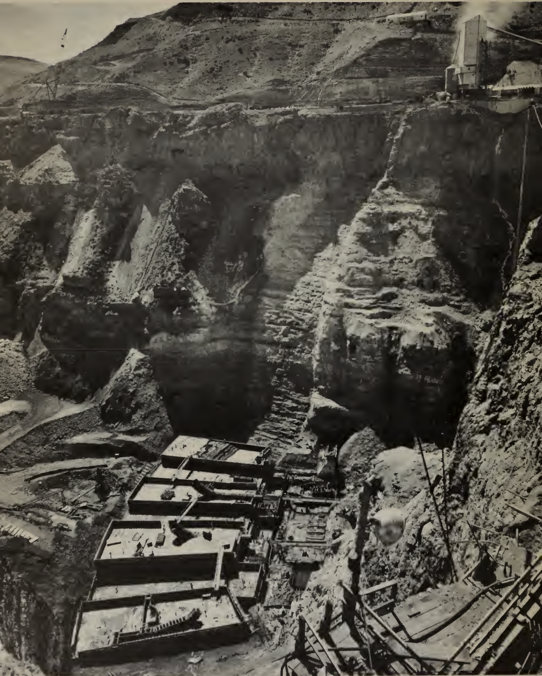
Yellowtail Dam begins to rise from the floor of the Bighorn Canyon in southeastern Montana. At the end of the fiscal year the average height of the structure was about 65 feet; when completed it will be 520 feet high.
