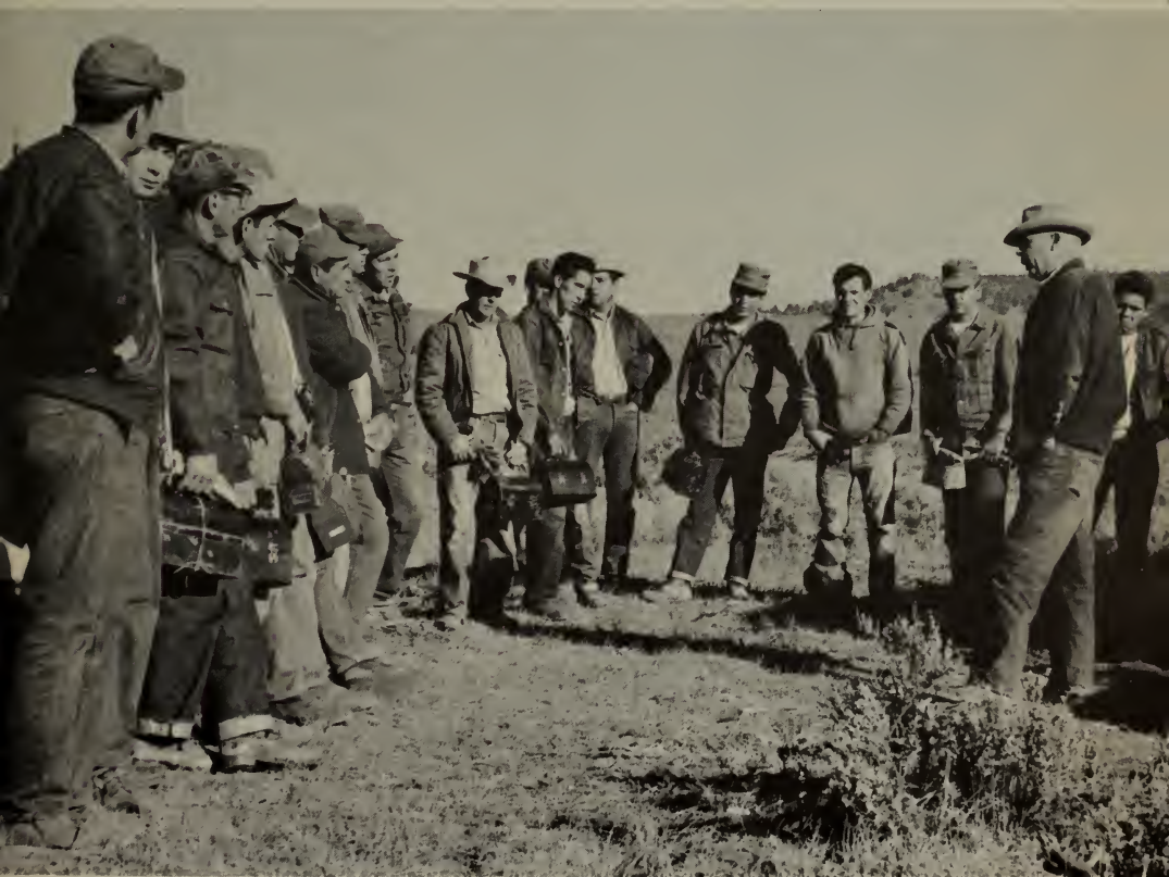
The Bureau of Land Management was one of the first Federal agencies to begin construction projects under the accelerated public works program. New employees, hired under the program, get safety instructions on their first day at work on the Rio Grande Gorge in New Mexico.
