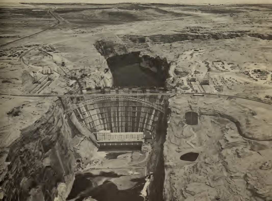
Beginning of work at Glen Canyon damsite, Arizona, in November 1957 can be seen in the above upstream view of the Colorado River. The aerial view of the damsite below in May 1963 shows the dam, powerplant and other works close to completion. Nearly 2 million acre-feet of water have been stored as Lake Powell starts to fill behind the dam.
