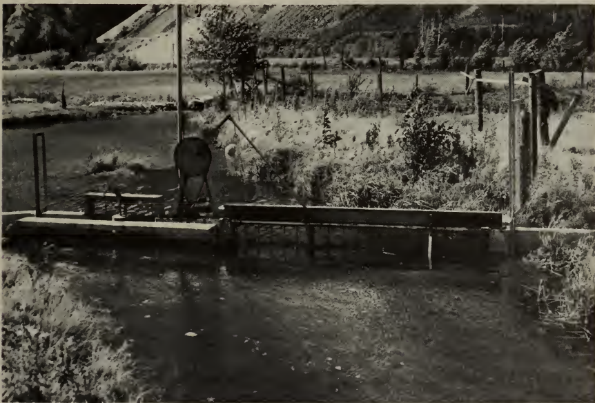
This fish screen prevents entry of young fish into an irrigation diversion on the North Fork of the Salmon River near Salmon, Idaho, where they soon would be stranded and die.— Courtesy Idaho Department of Fish and Game.
