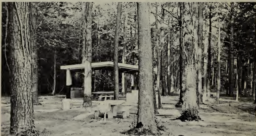
Under the accelerated public works program, new recreation facilities such as this picnic shelter with tables and charcoal grills were provided on Blackwater National Wildlife Refuge.
