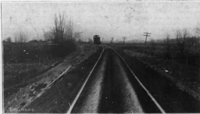
Fig. 1.—Ballast Dumped.
