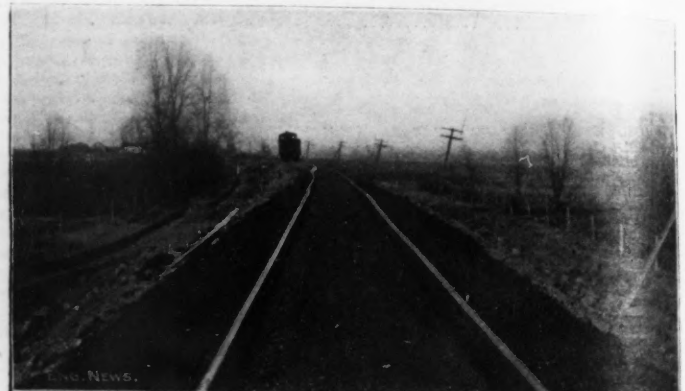
Fig. 2.—Ballast Plowed.
