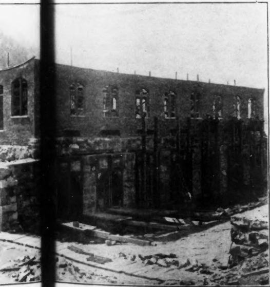
FIG. 6. VIEW OF POWER HOUSE UNDER CONSTRUCTION, FROM HEAD RACE SIDE.
