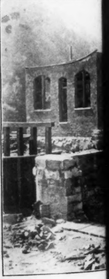
FIG. 6. VIEW OF DAM
