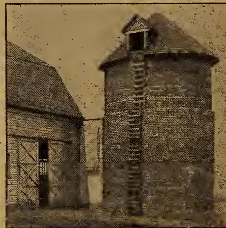
Brick is a good standard silo material. Note the thinner wall at the top
