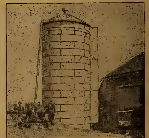
Metal silo made of pure anti-corrosive iron are not short-lived
