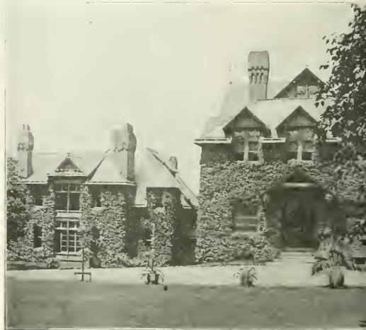
Administration House and Powers' Cottage, Hospital for Diseases of the Lungs, Chestnut Hill.
