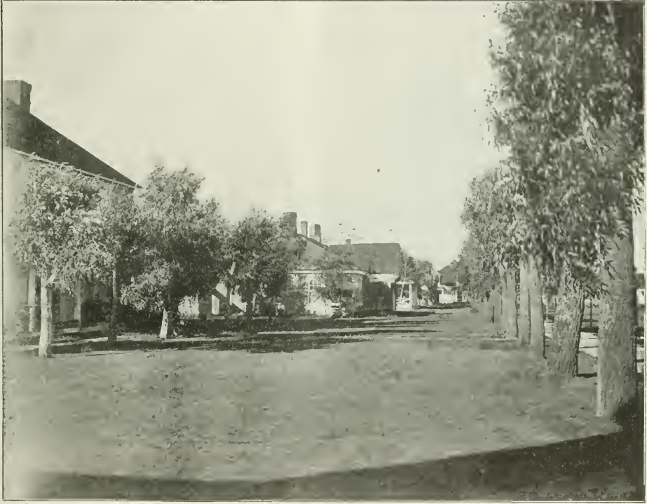
Fig. 4.—Showing Officers' Quarters. Fort Stanton, New Mexico.
