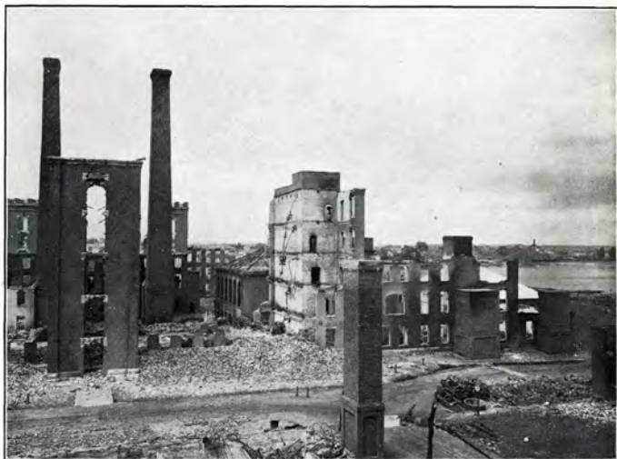
General View of Ruins. From roof of No. 1 Store House looking northeast.
