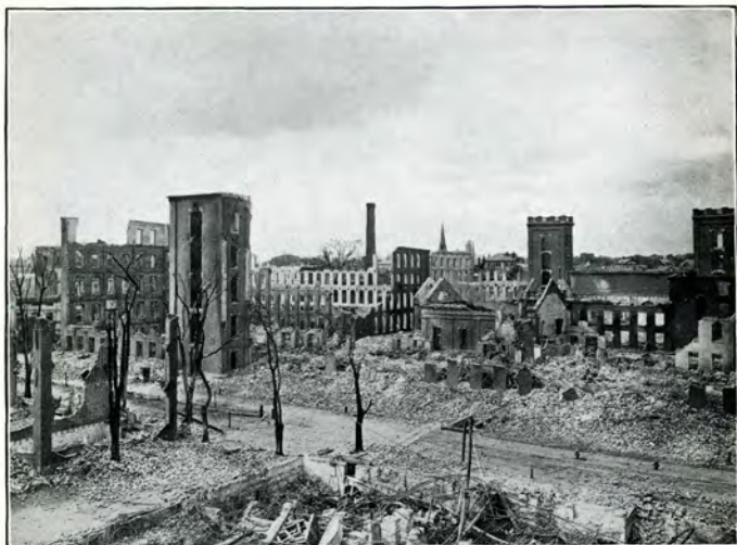
General View of Ruins. From roof of No. 1 Store House looking northwest.
