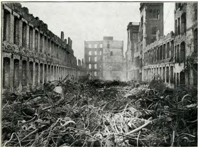
Interior of No. 2 Mill, showing wreckage of machinery.
