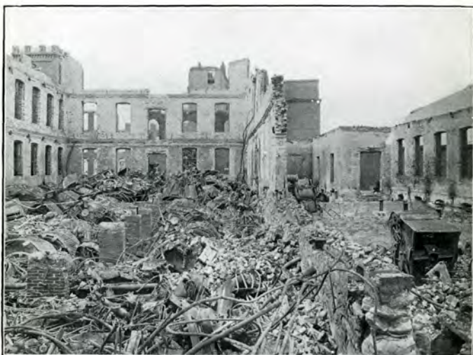
Wreckage. Interior No. 1 Picker House.
