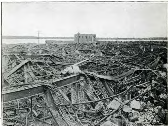
Wreckage. Floor beams, etc., No. 6 Weave Building.
