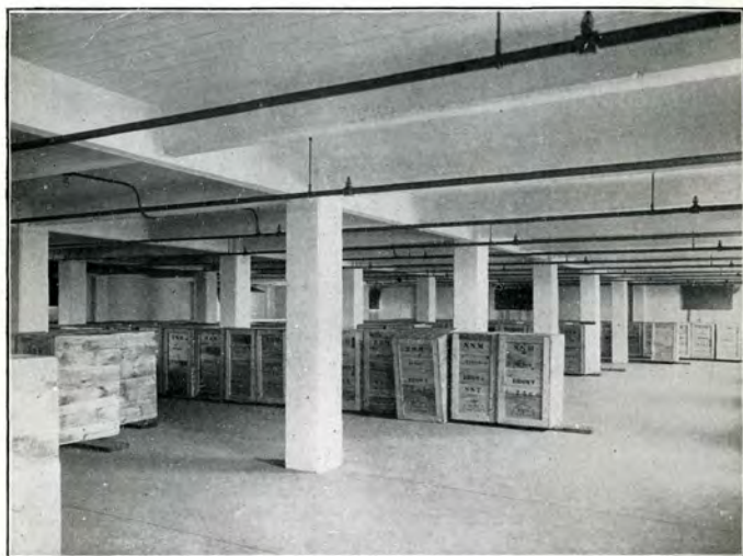
Interior of No. 1 Store House. Note perfect condition of building and contents.
