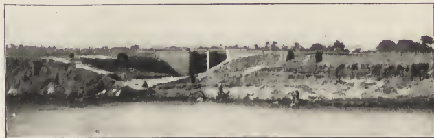
A Water Gate.
