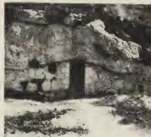
Entrance to King Solomon's Quarries.
