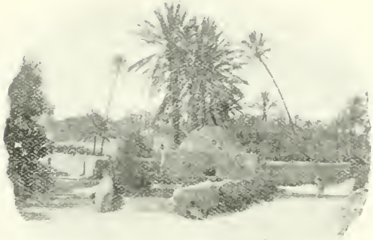
Junction of Roads outside Tripoli.
