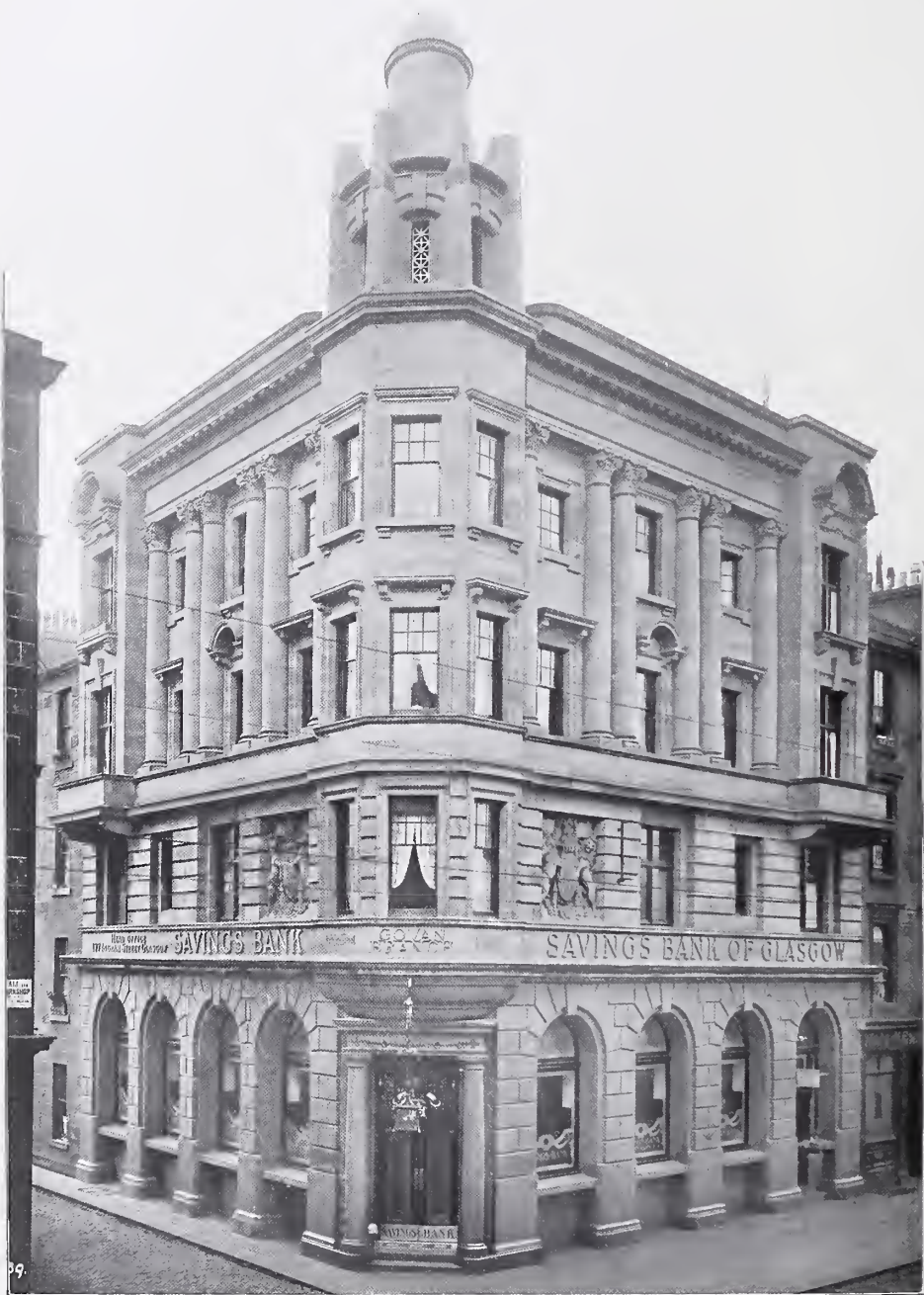
791. Savings Bank of Glasgow, Govan Branch, ERIC A. SUTHERLAND, Architect. Mason: G. Barlas and Co., 13 Ruthven Street, Hillhead, Glasgow. Joinery: John Cochrane, 58-70 Dobbies Loan, Glasgow. Marble: Galbraith and Winton, 185 St. Vincent Street, Glasgow. Heating: Cameron and Co., Glasgow.
