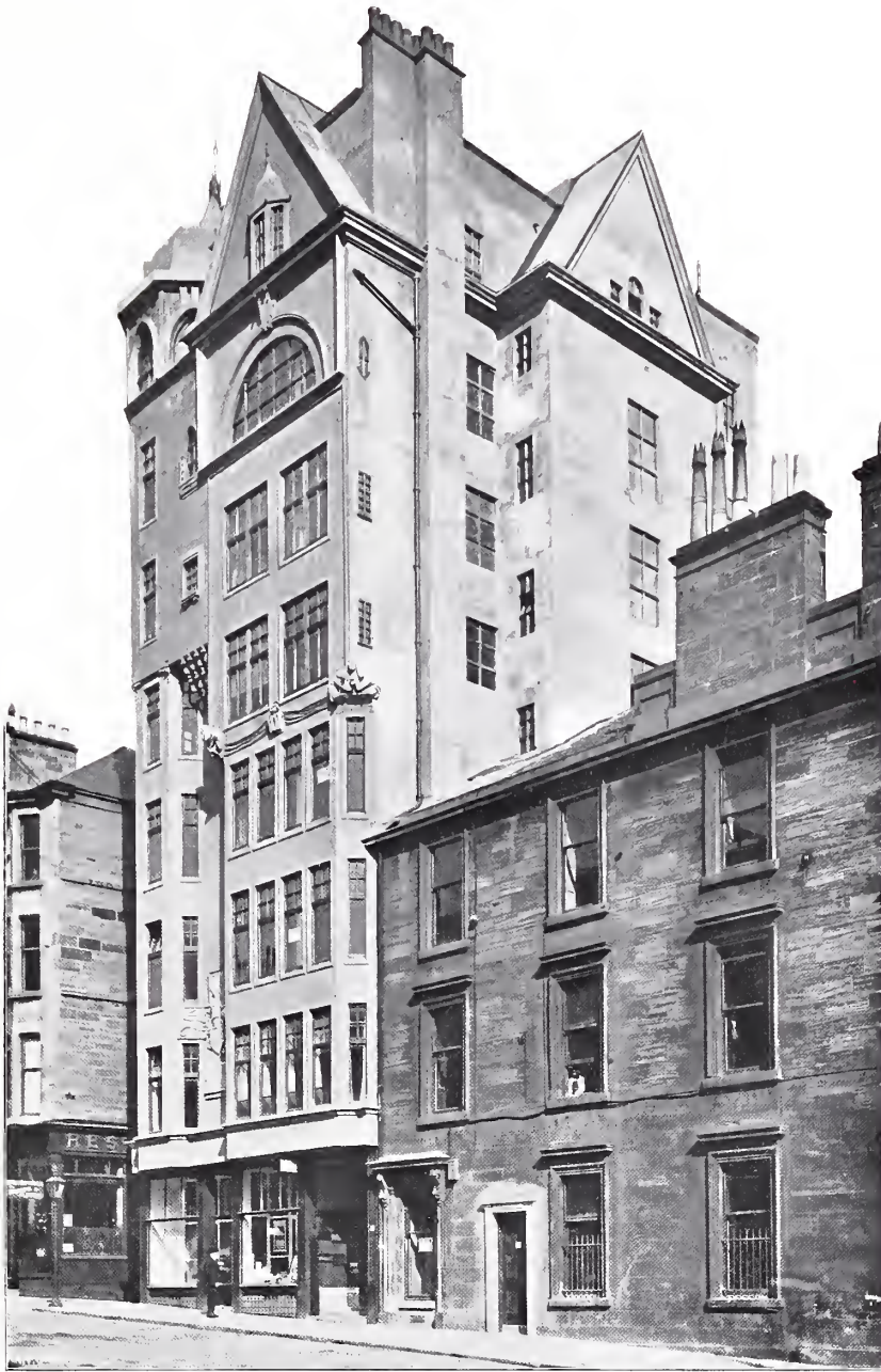
795. Lion Chambers, Hope Street, Glasgow, SALMON AND SON AND GILLESPIE, Architects. Ferro Concrete: The Yorkshire Henebique Contracting Co., Ltd., Leeds. Joinery: Geo. Laird and Son, 10 Ann Street, Bridgeton, and 183 Bath Street, Glasgow. Elevators: A. and P. Stevens, 179 St. James' Road, Glasgow.
