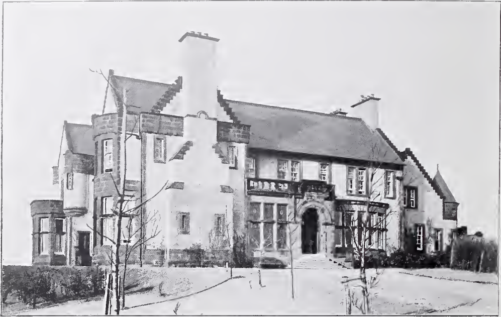
787. Carnbooth, Busby, N.B., ALEXANDER CULLEN, Architect. Contractor: Robert Aitkenhead and Sons, Higher Blantyre.
