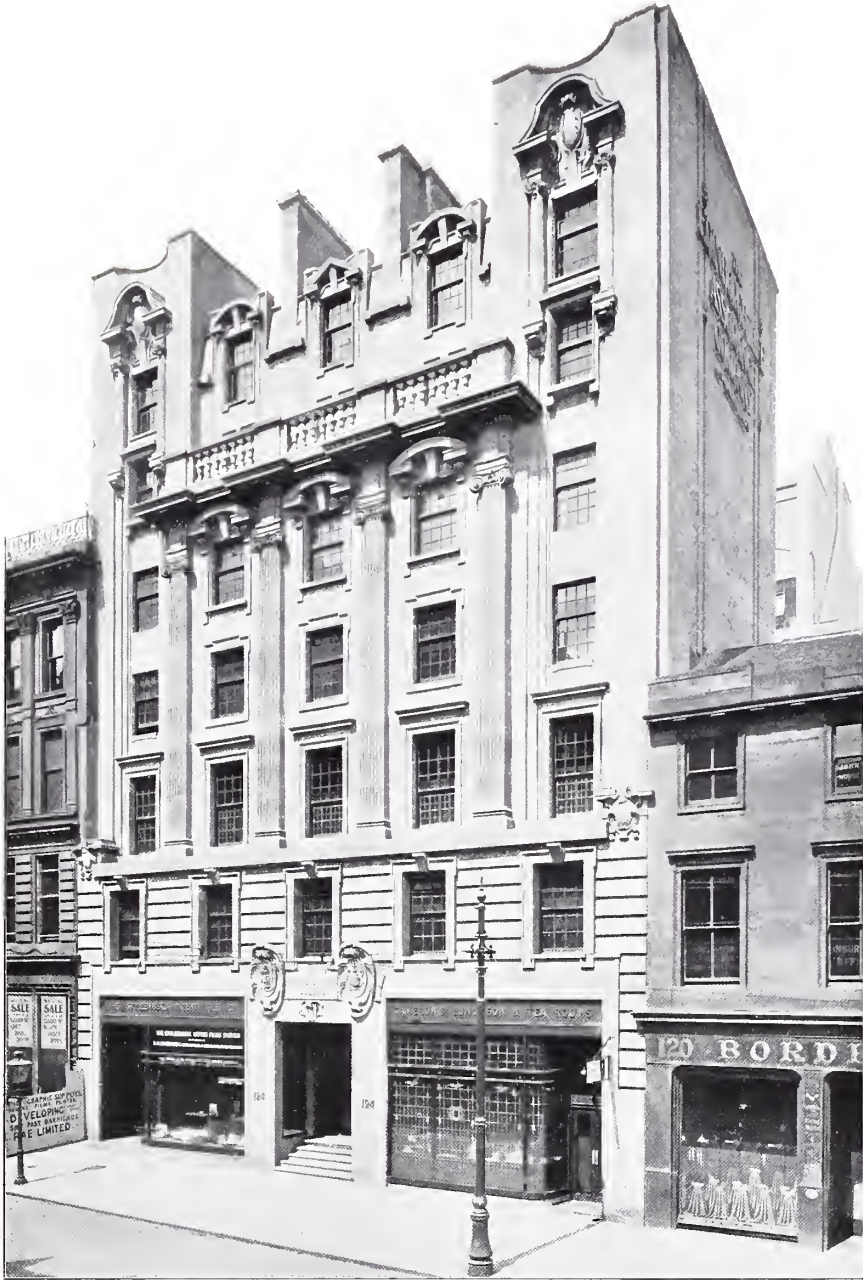
776. Edinburgh Life Assurance Company , JOHN A. CAMPBELL, Architect. Mason: Morrison and Mason, Polmadie, Glasgow. Fireproof Flooring: D. Ferguson and Co., Glasgow.
