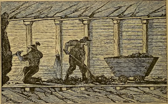
Longitudinal View of Timbered Level.
