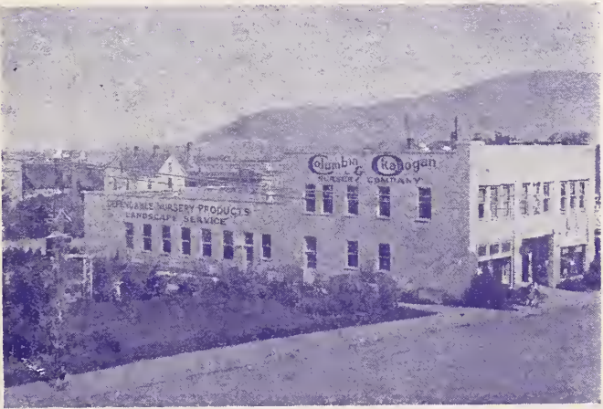
Office and Packing House Located At Wenatchee, Washington
