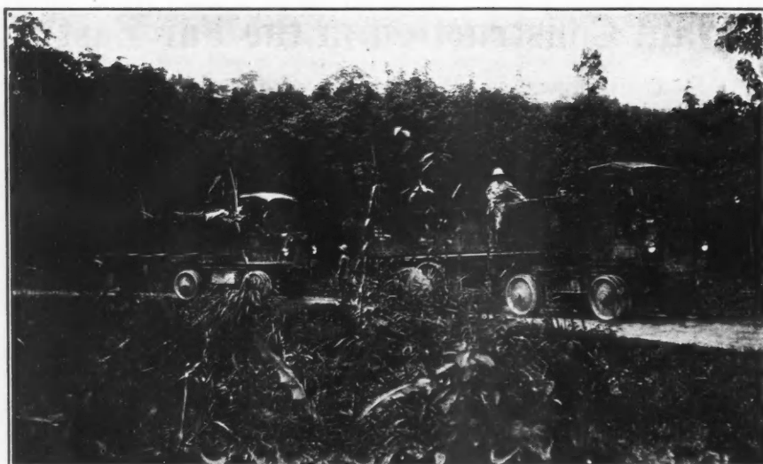
Transporting spud casing for dredge
