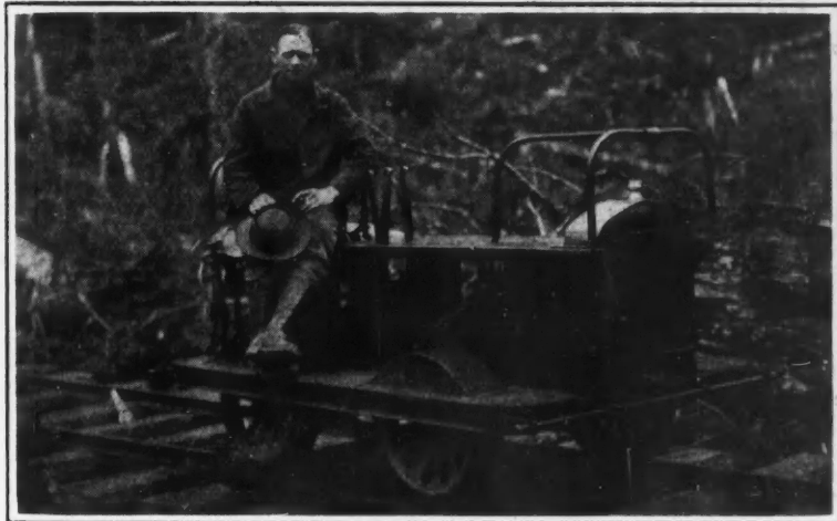
One of the locomotives used to haul supplies over the Dolly Varden narrow-gauge railroad
