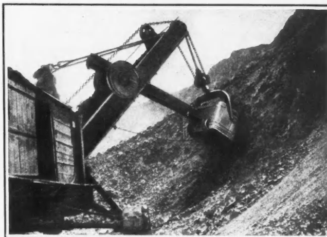
Caterpillar tractor shovel at Utah Copper open pit
