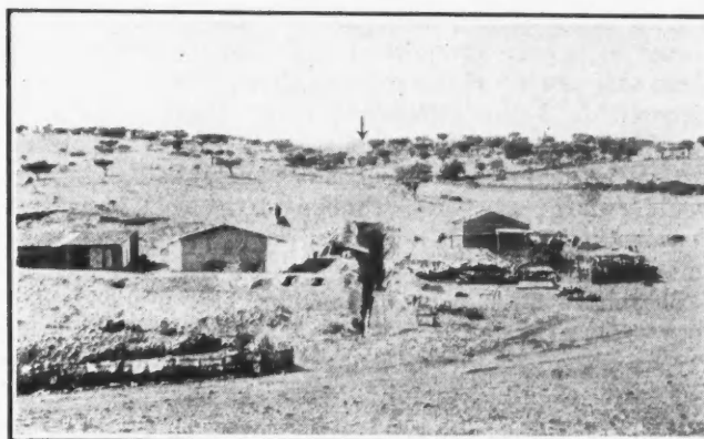
Bunk houses and portal of the Vieros mine
