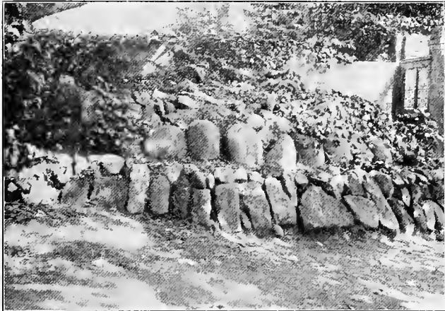
8. Garden rockery, illustrating some bad points of construction (page 36).
