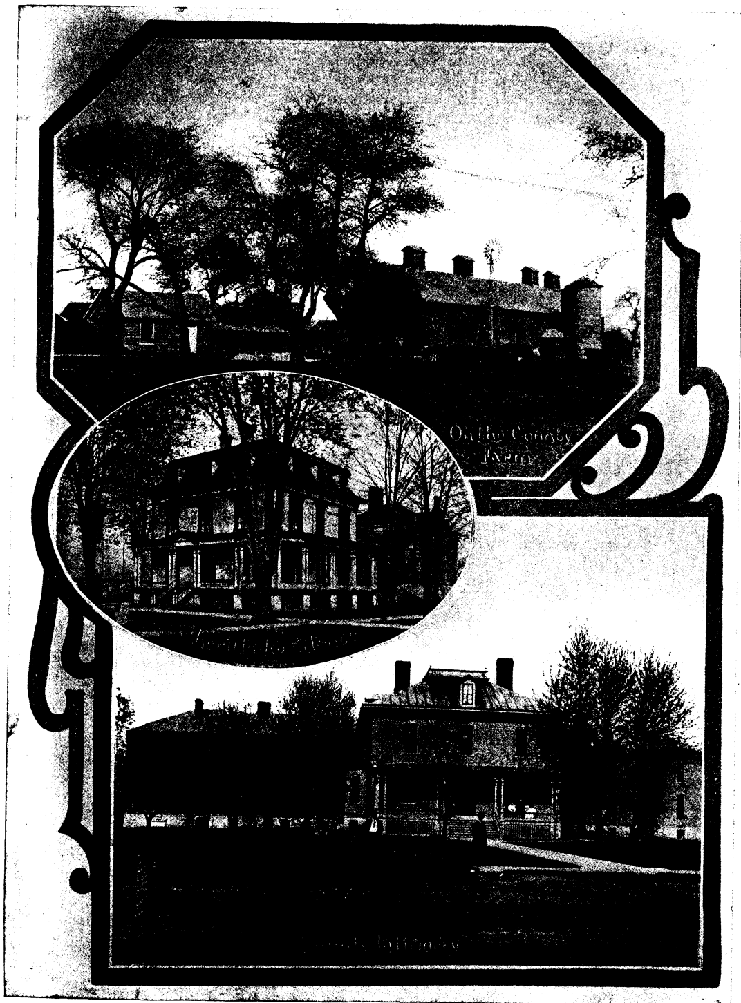
MONROE COUNTY BUILDINGS
