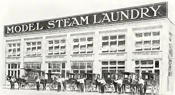
OUR NEW PLANT
