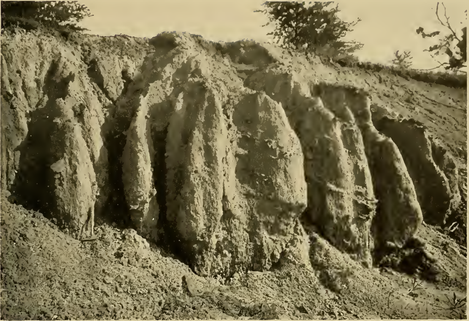
FIG. 1.—VIEW SHOWING EROSION OF ARUNDEL CLAYS, HARTKE IRON MINE NEAR HANOVER, HOWARD COUNTY.
