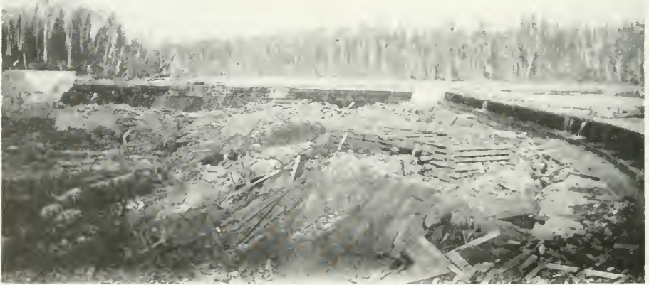
Concrete dam replacing timber structure at Sandy falls
