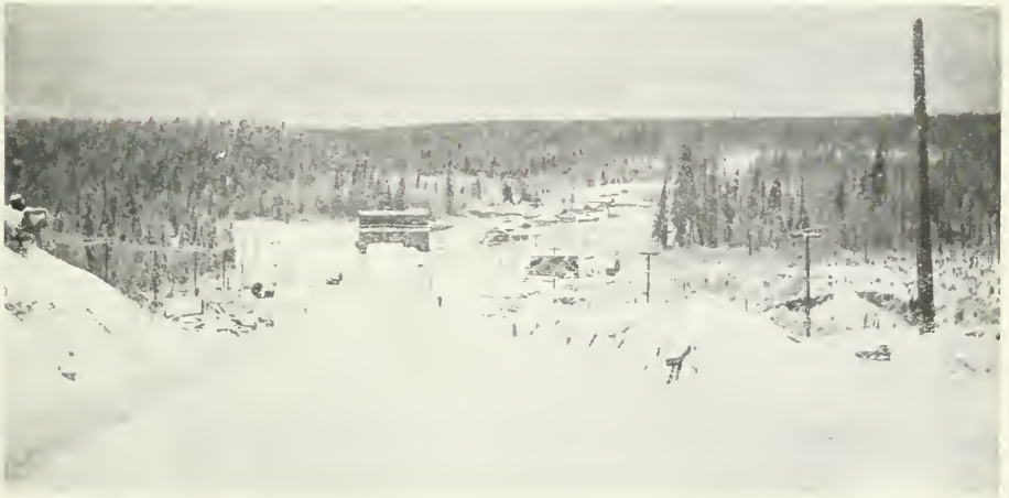
View of Wawaitin power house looking down the line of eight foot penstocks (covered). A new nine-foot wood stave penstock has been added recently
