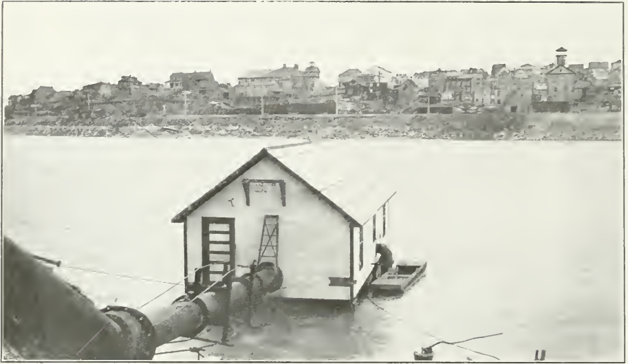
Cobalt Lake before dewatering
