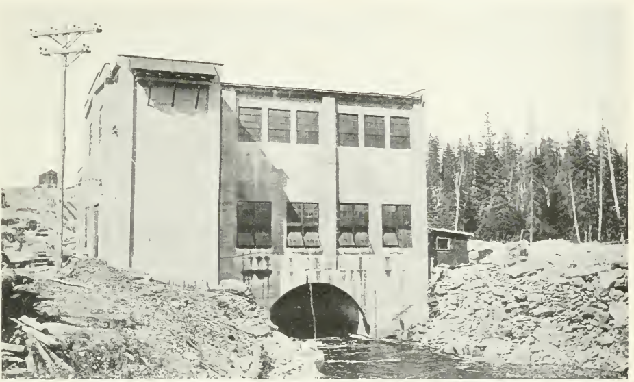
Power house, Wawaitin falls, Mattagami river, township of Thorneloe. Eight-foot penstocks lead from the surge tank at the crest of the hill to the power house
