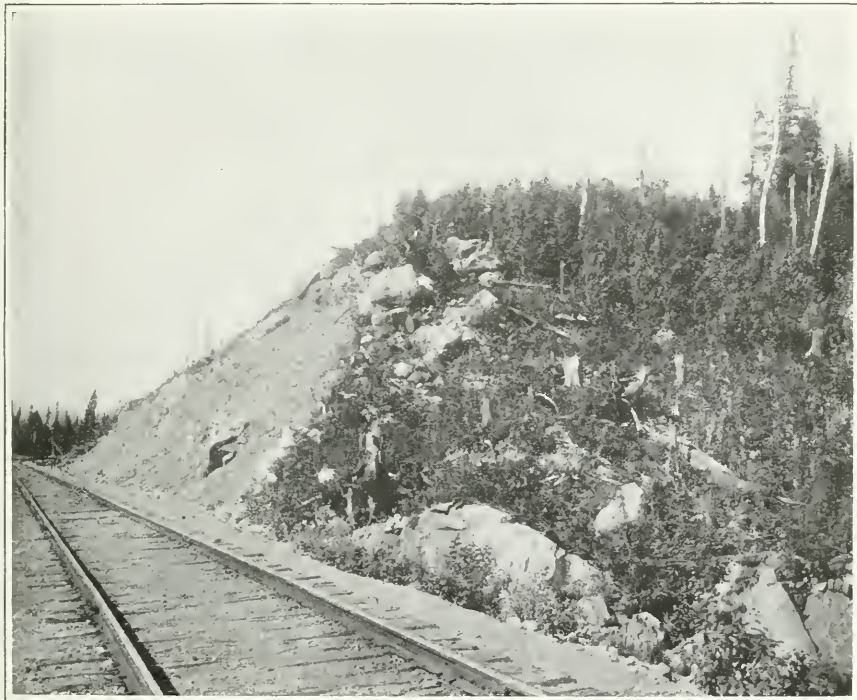
Fig. 6—Partially decomposed pre-Cambrian rock in place, showing angular fragments in the railway cut near Mile 162, A.C. and H.B. Railway
