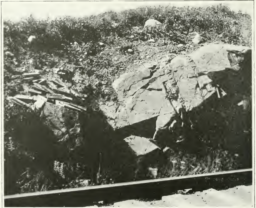
Fig. 8—Partially decomposed Keewatin rock overlying polished surface of Keewatin rock. The polishing is probably due to creeping of the overlying material.
