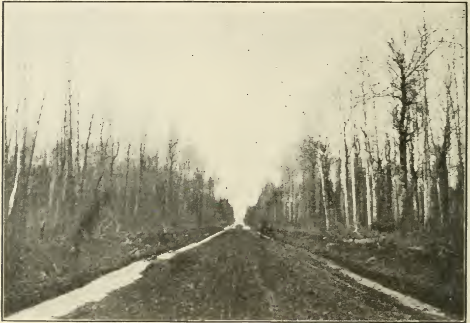
New road under construction in the Rainy River Valley.
