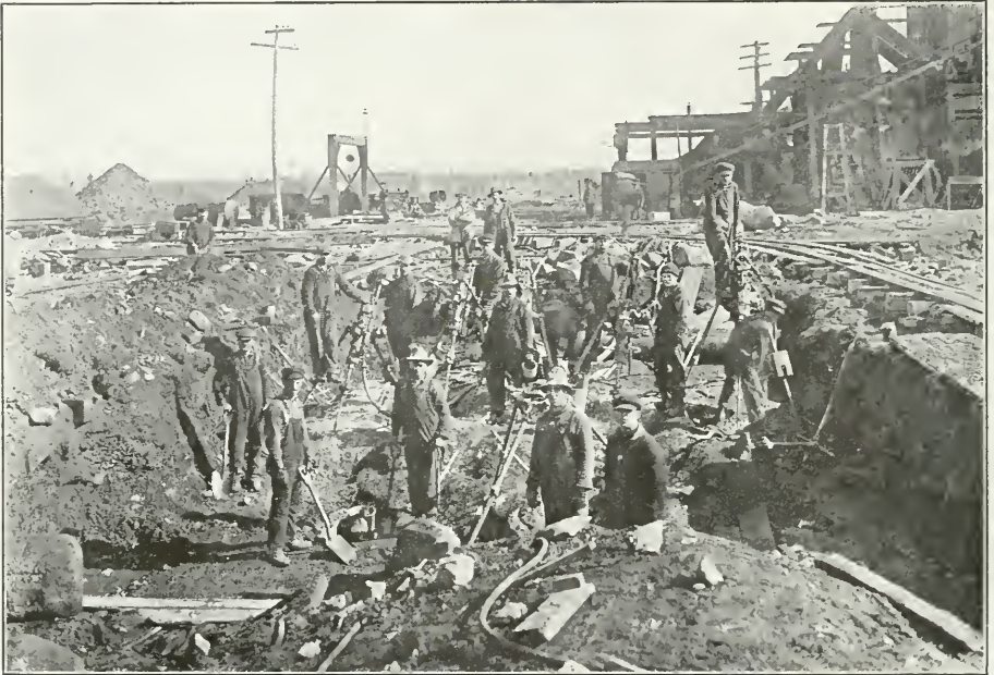
Starting 5-Compartment Shaft at Creighton Mine.
