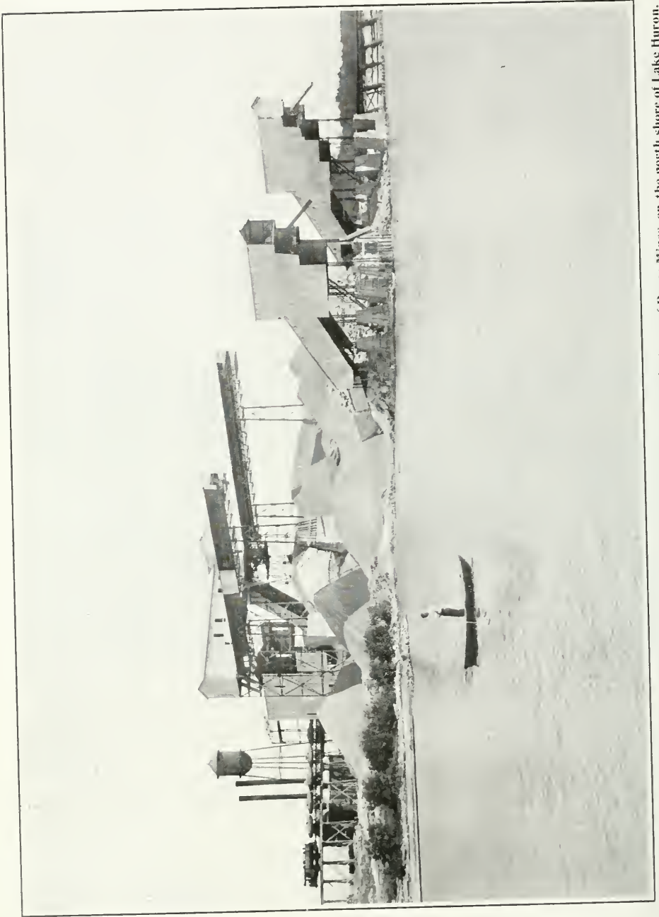
Fig. 12—Plant and stock piles of the Martin International Trap Rock Company at the town of Bruce Mines, on the north shore of Lake Huron. The crushed rock is used in road making
