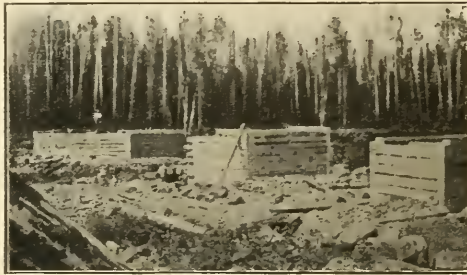
Constructing bridge across Mattawishquia River near Hearst.
