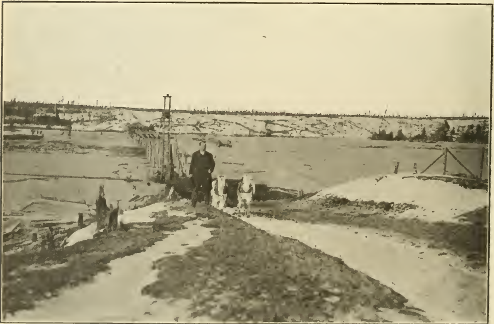
Constructing the Matheson Bridge, 650 feet long.
