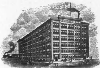
FACTORY 132 ND TO 133 RD ST. & BROOK AVE
