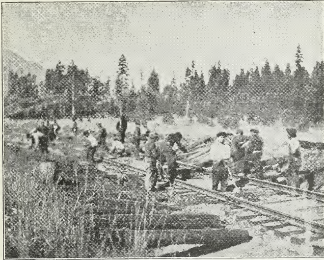
FIG. 12.—Fully half of the annual production of railroad ties is used to replace ties decayed in service. Less than half of all ties installed are now treated with preservatives. The possible saving of wood by this practice is enormous
