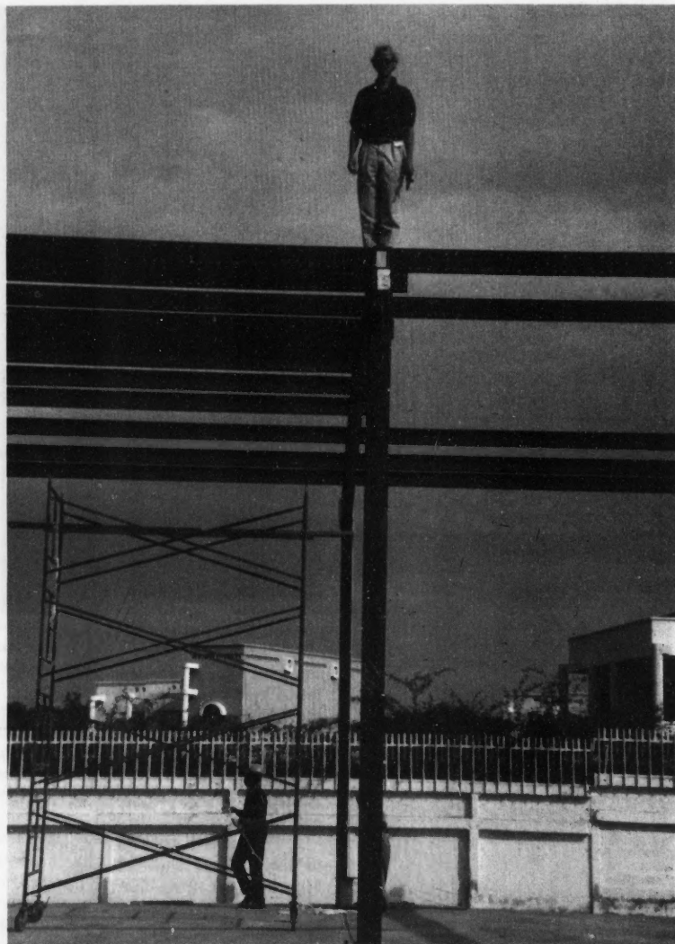
The author (top) at the construction site in Mauritania.
