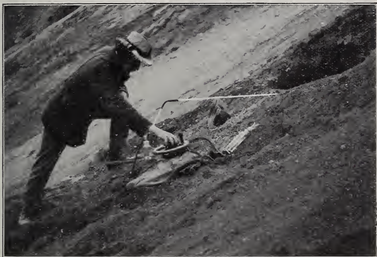
FIG. 7. Collecting gases from a fumarole at a temperature of 438° C.
