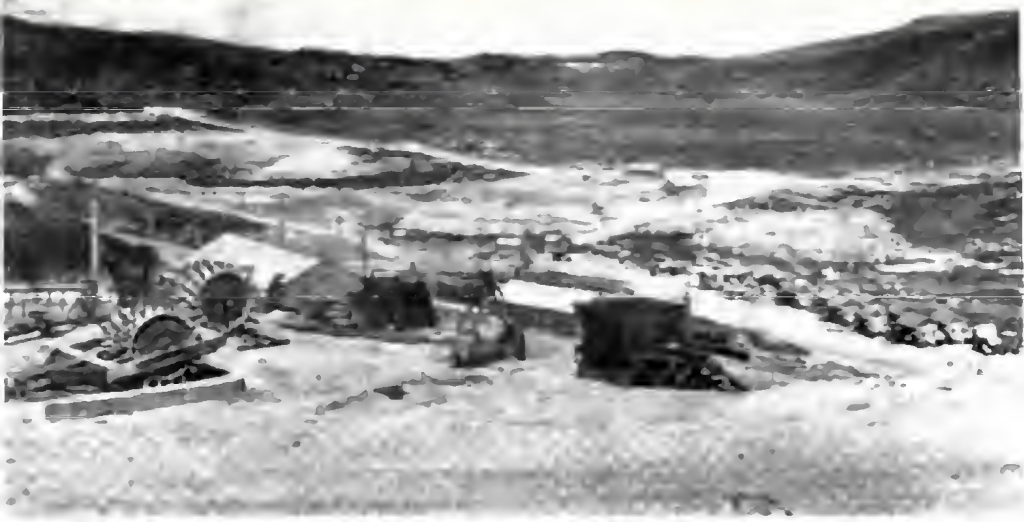
Earthworks and Machinery in Rocky Valley
