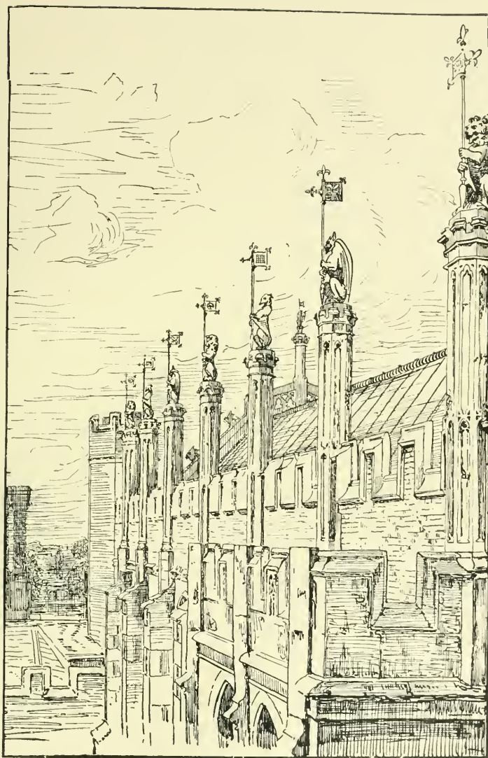
Parapet of the Great Hall as seen from the Roof.
