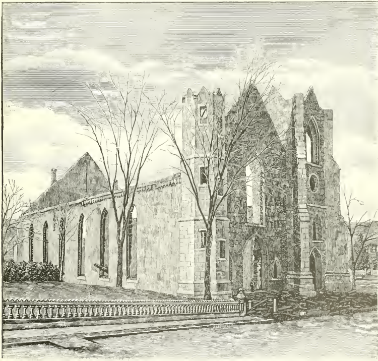
ST. JOHN'S CHURCH, AFTER THE FIRE OF DECEMBER 24, 1868.
