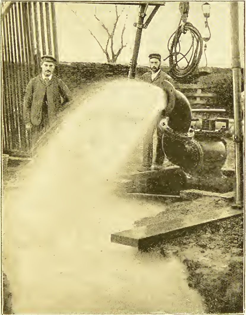
FIG. 9.—Illustrates the overflow from an Artesian well recently bored at Bourn, Lincolnshire, by Messrs. C. Isler and Company, for the supply of the town of Spalding. The overflow is at the rate of about 5,000,000 gallons per day, and is probably the most prolific underground spring yet tapped in England. The boring is only 134 feet deep.
