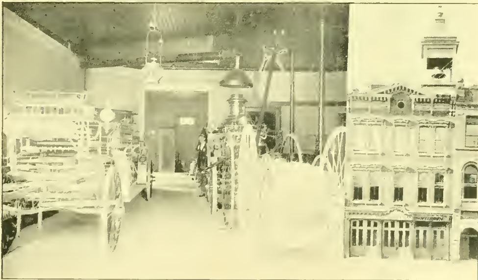
Harris, Photos. HEADQUARTERS OF THE CORTLAND FIRE DEPARTMENT.
