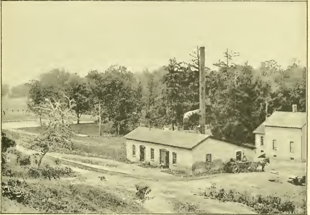
THE CITY WATER WORKS.
