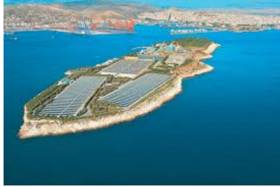
Figure 15. Wastewater Treatment in Psytalia Island, Greece
