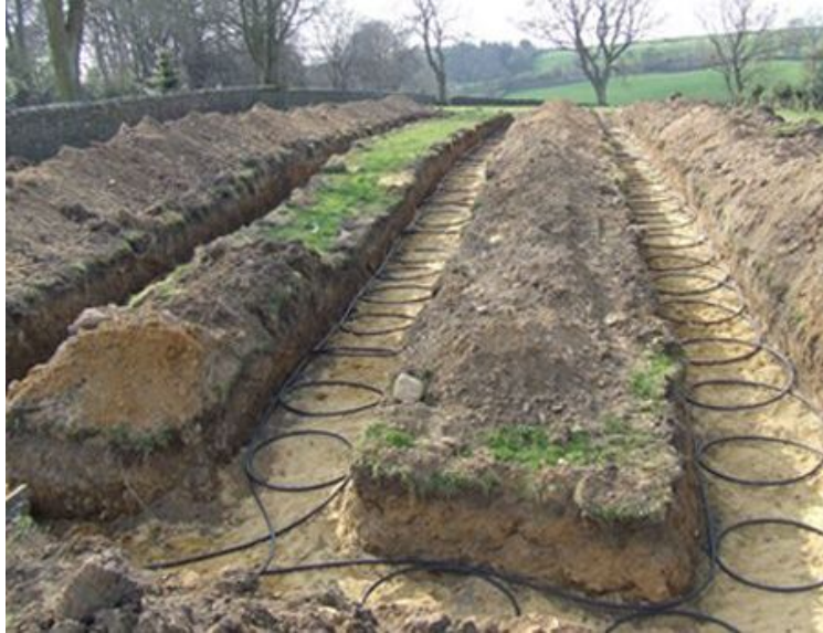
Figure 8. Part of Installation of a Geothermal Heating Pump
