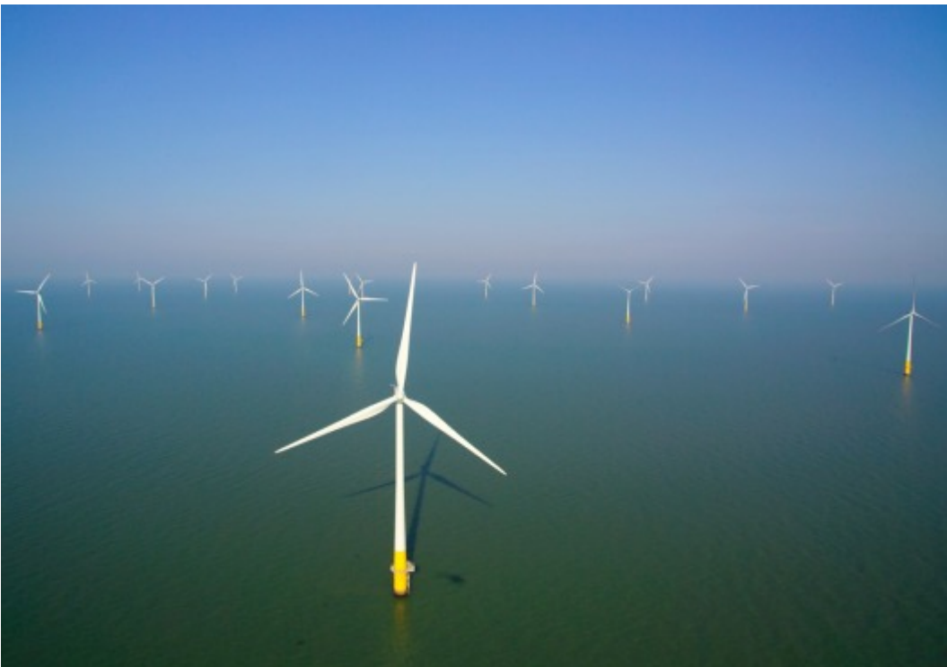
Figure 3. Offshore Wind Farm
