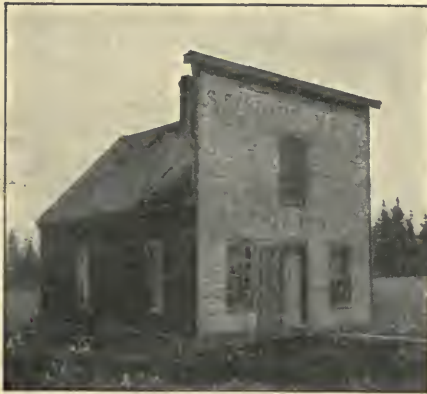
"The first frame structure"
