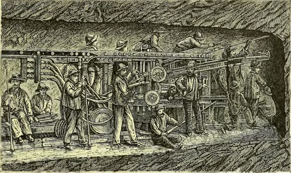
Fig. 1. Bohrmaschine, System Comellier.
